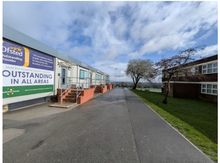
Photo 2 - View of Modular building adjacent to main school building
