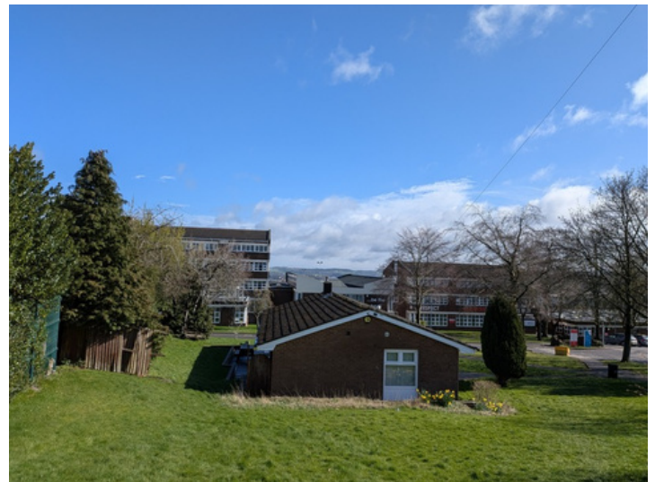
Photo 12 - View of entrance to Moor End Academy (modular units not visible)
