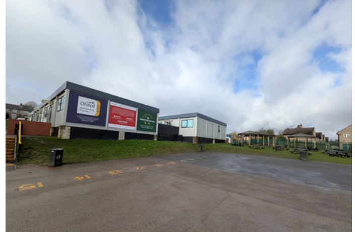
Photo 6 - Rear view of modular buildings from playground and neighbouring residential property
