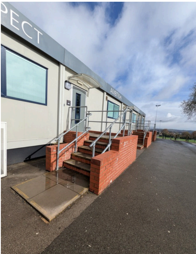
Photo 3 - Stepped entrance into portakabins (bricked in - demonstrating permanence)
