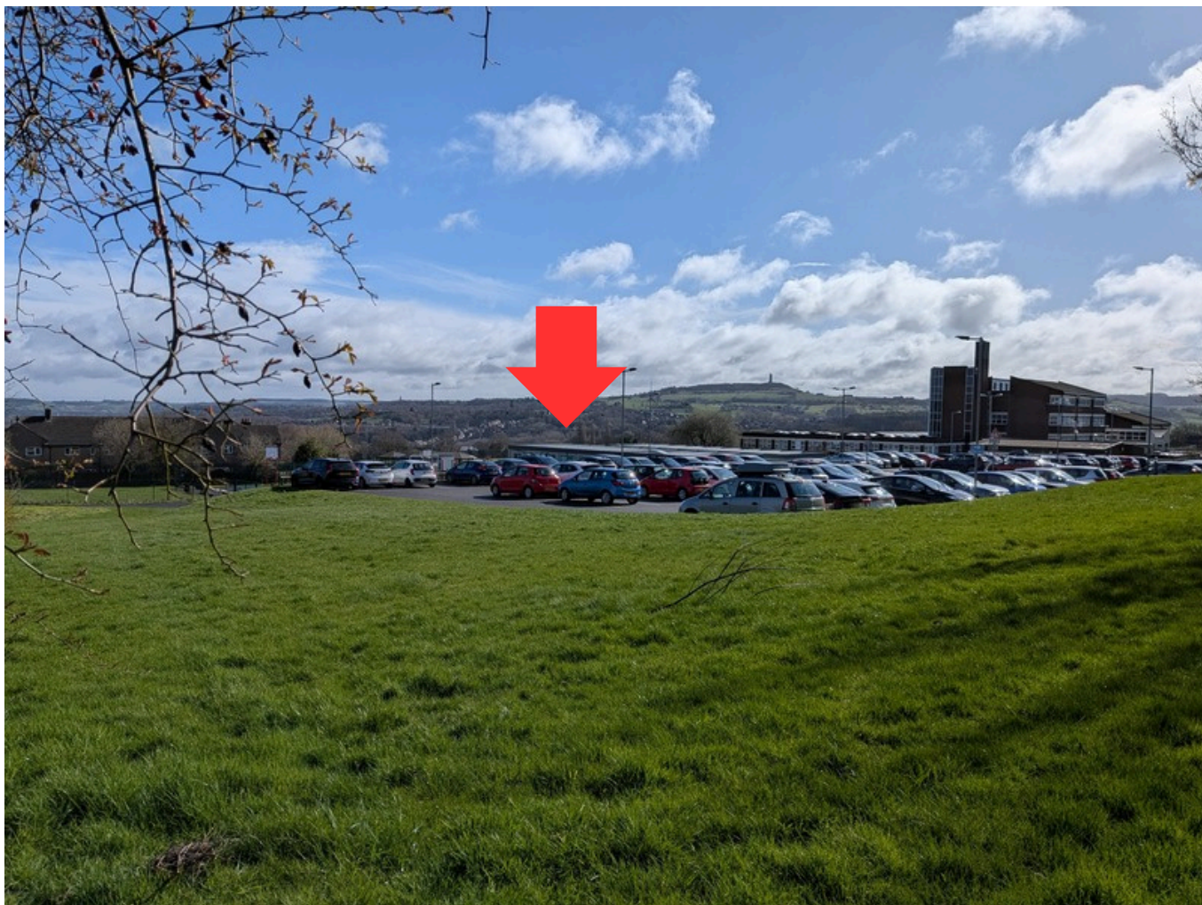
Photo 15 - View of modular buildings from within the school boundary fence. The 2no. modular buildings (highlighted with a red arrow) are positioned below the existing car parking and are visually contained by the surrounding built form. By virtue of their single-storey scale and modest height, they remain clearly subservient to the main school building and do not result in any material harm to the character or appearance of the area.
