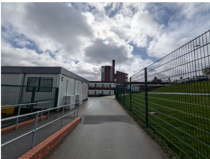
Photo 9 - Single height modular buildings (subservient to main school building in background)
