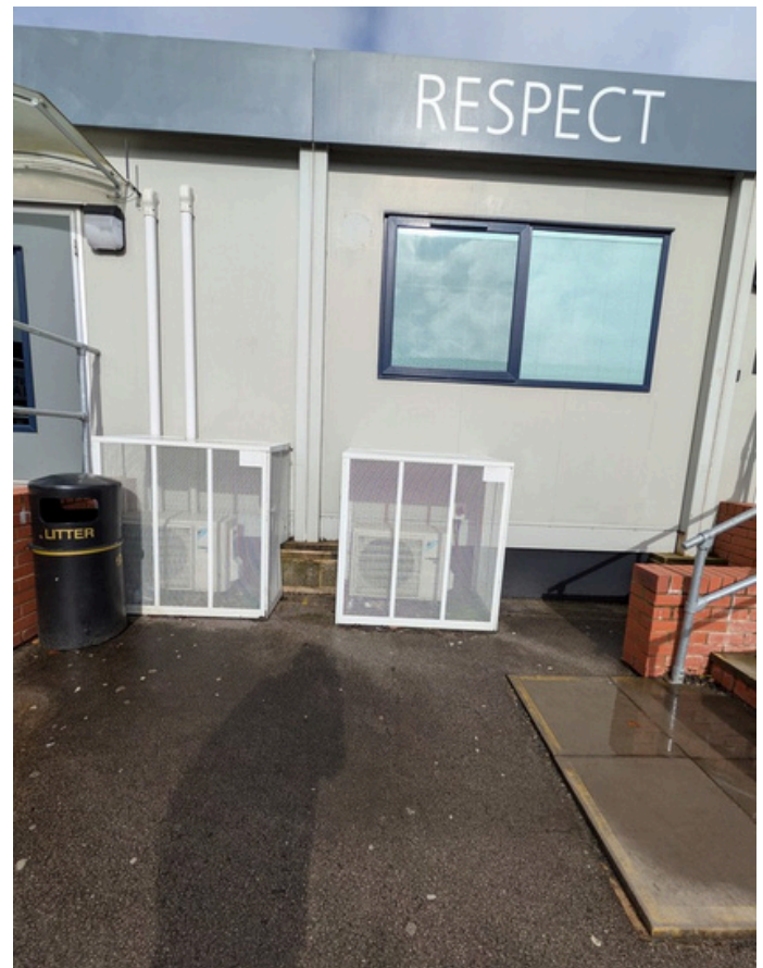
Photo 4 - Modular construction foundations and AC units (services) demonstrating permanence
