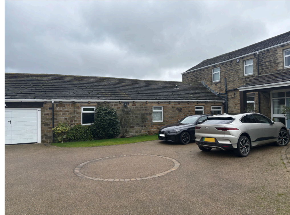
Figure 2 – Single storey section to house the new entrance with oak frame canopy
