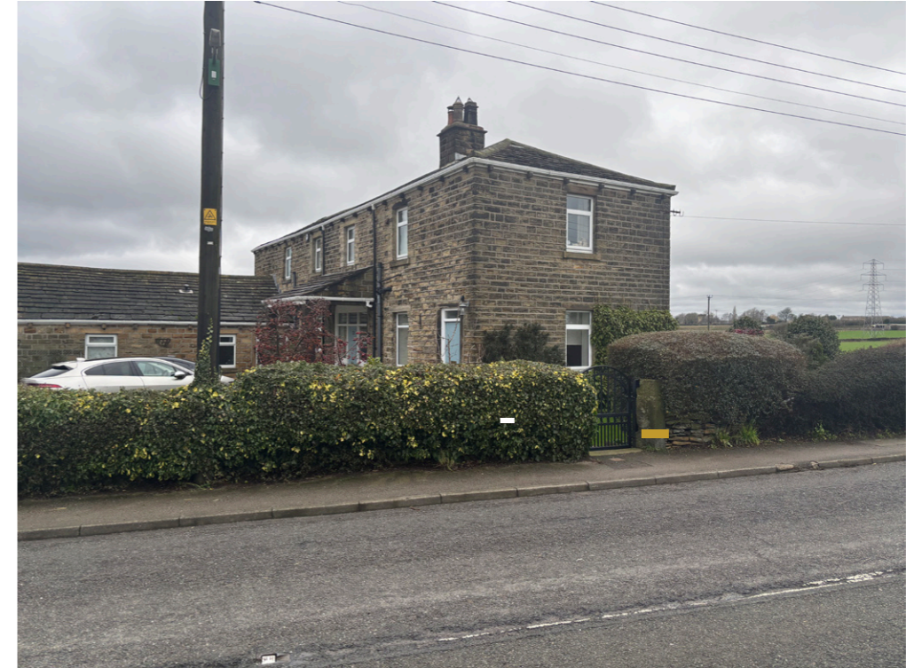
Figure 6 – Existing door canopy to be removed and door entrance to be replaced with feature arched window
