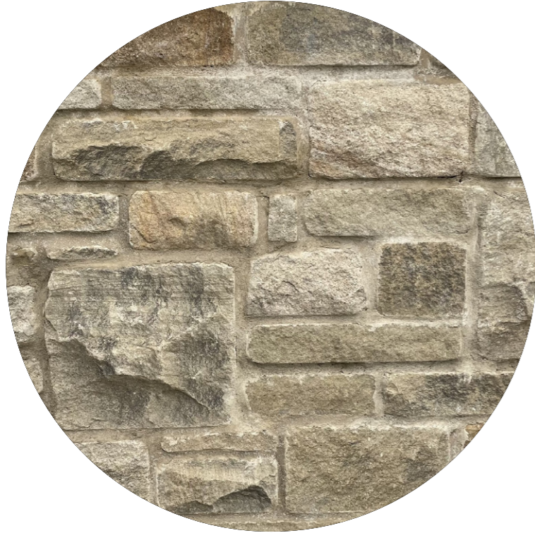
Natural stone walling to match existing
