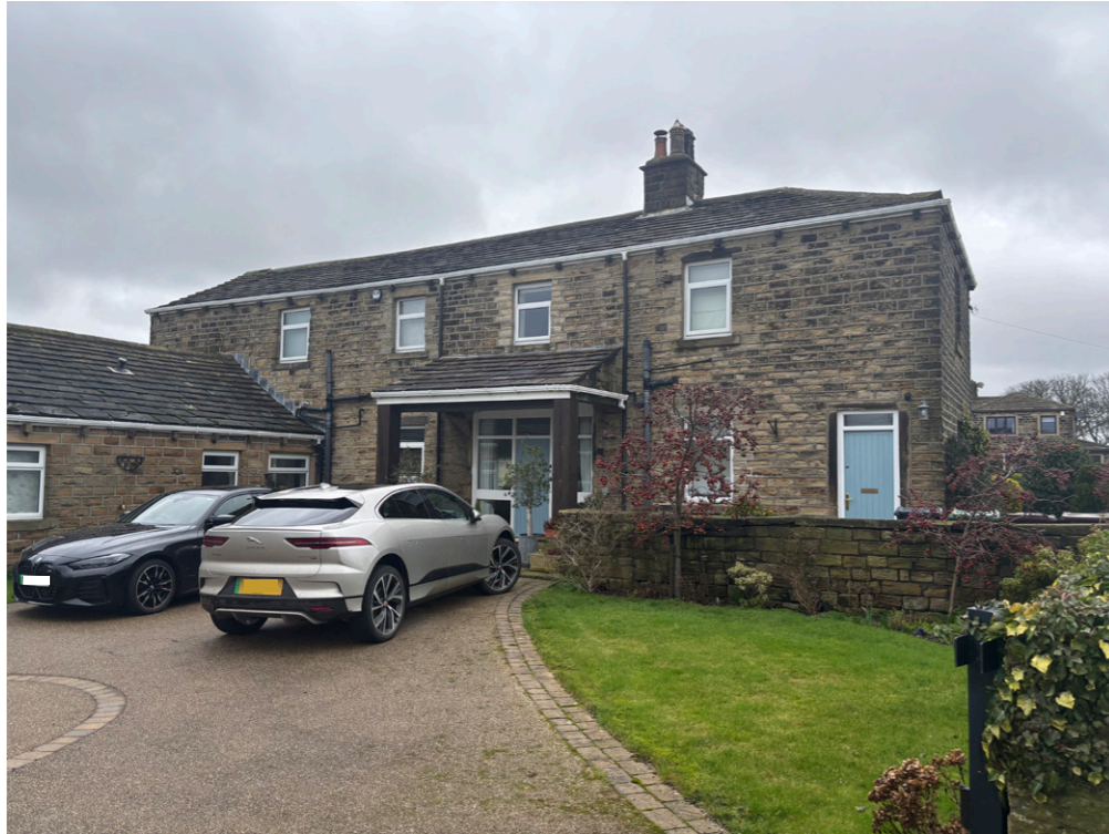
Figure 1 – Photo of existing front door and two storey section of the house
