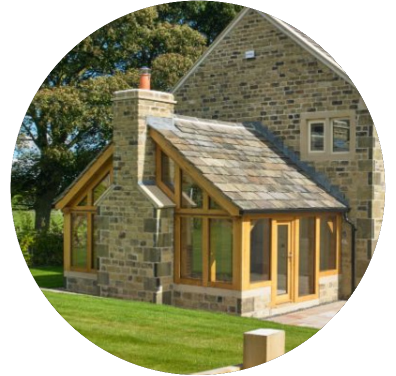
Oak frame features including the canopy / posts and rear extensions feature truss, terrace and posts
