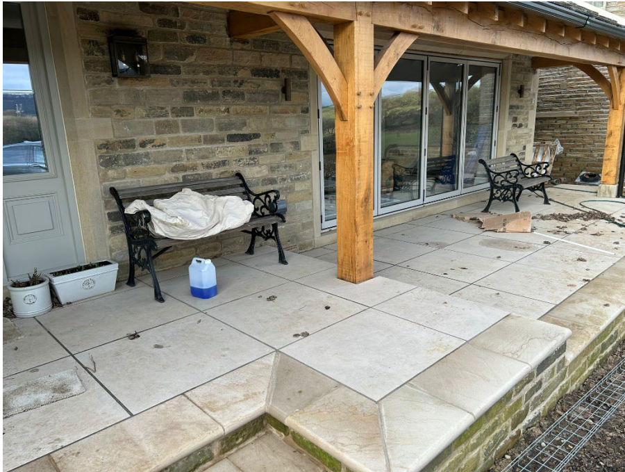
Photograph 1: External stone paving placed in area of WS02.
