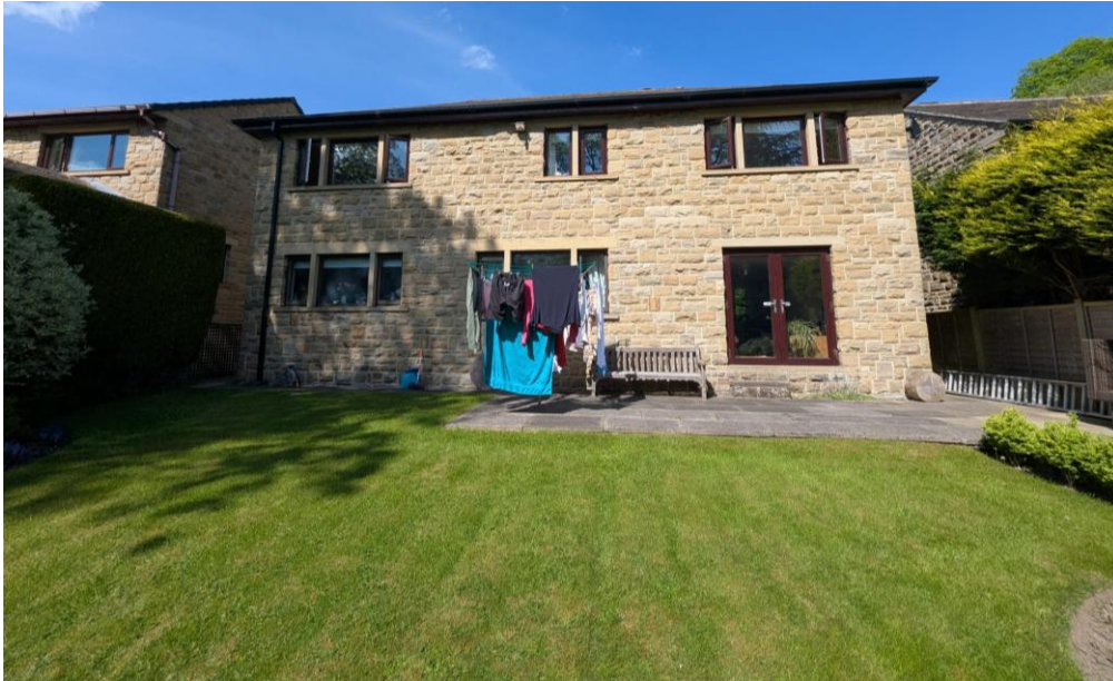
Existing rear of the property
