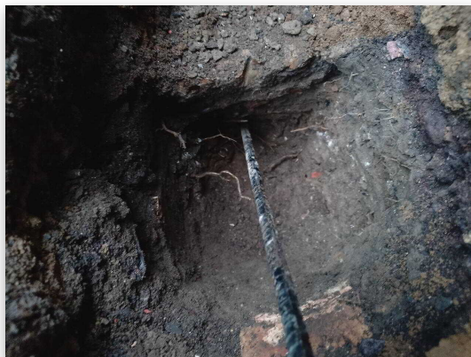
Fig 1.2: Trial Hole 1 Footing
