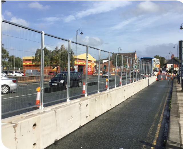
TVCB's with fence securing highway
