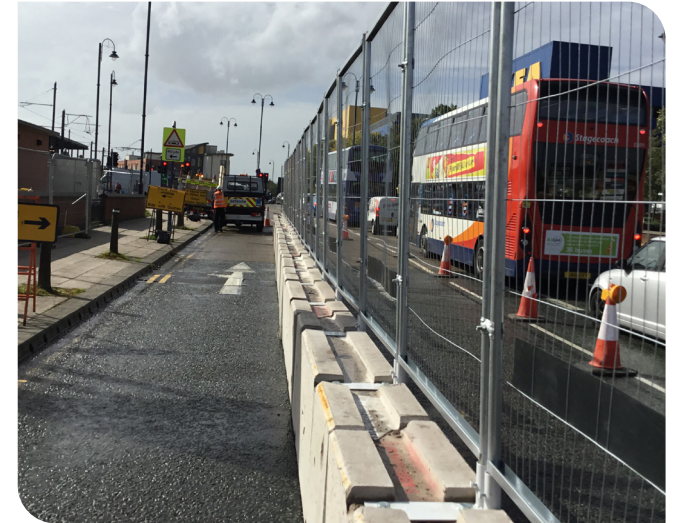
TVCB's creating safe zone for workers
