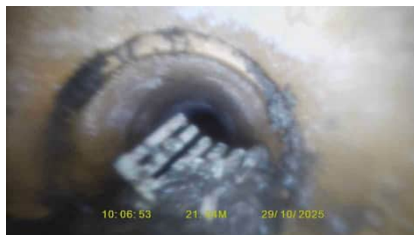
S15X_abfa47d0-0b22-45b1-b541-ebcfbccd7dea_20251120_1 13018_978.jpg, 00:01:43, 21.70 m Survey abandoned, Silt & objects
