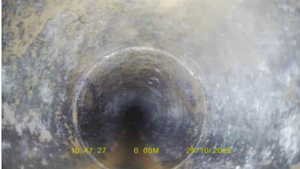
FW13X_120424f2-95b7-4a33-b99d-3f17215606e5_20251120_123632_215.jpg, 00:00:00, 0.00 m Start node, inspection chamber, reference: FW12
