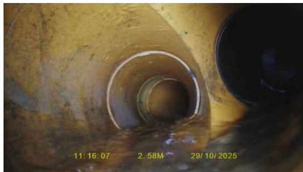
S21X_64fa01cf-0235-4dbd-99d6-82904f55b836_20251120_1 31551_306.jpg, 00:00:12, 2.60 m Junction at 3 o'clock, 100mm dia
