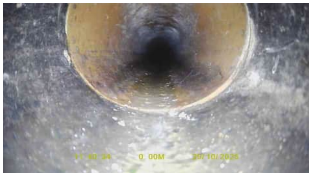
F26X_cd651f74-8b93-40b2-9cff-cec93c3565f6_20251120_132755_150.jpg, 00:00:00, 0.00 m Start node, inspection chamber, reference: FW13
