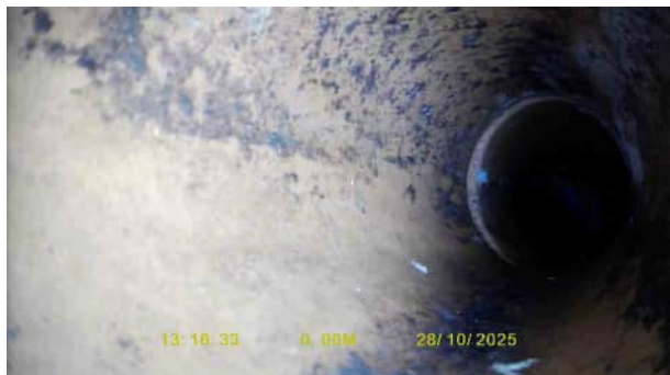
FW4X_6a979b06-3db2-46b8-920d-588961a563c6_20251111_143602_325.jpg, 00:00:00, 0.00 m Start node, inspection chamber, reference: FW3
