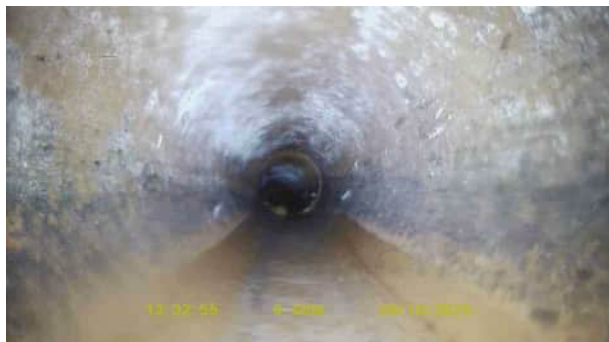
FW5X_63541612-0bb5-4a39-b3e8-42141940315e_20251119_141452_504.jpg, 00:00:00, 0.00 m Start node, inspection chamber, reference: FW3
