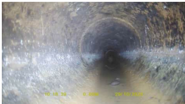
FW11X_3dda44b6-7823-4467-965d-606f375b9f11_20251120_113752_197.jpg, 00:00:00, 0.00 m Start node, inspection chamber, reference: FW10
