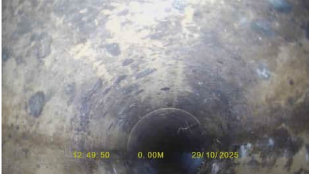
F30X_2214ed51-15aa-4e46-aab5-35143f1f0843_20251120_142439_476.jpg, 00:00:00, 0.00 m Start node, inspection chamber, reference: FW15
