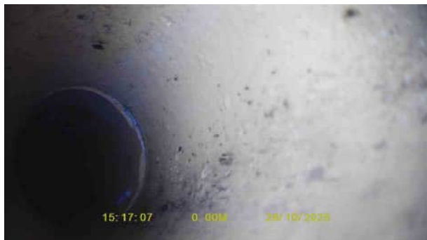
F17X_89a12d6c-1439-48ec-8b76-36ee0f1930c7_20251120_085611_524.jpg, 00:00:00, 0.00 m Start node, inspection chamber, reference: FW6
