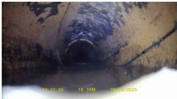
FW10X_69e5f6ae-08e1-45af-9fc6-638c67ddbe9d_20251112_102045_864.jpg, 00:01:39, 18.60 m Joint displaced, large
