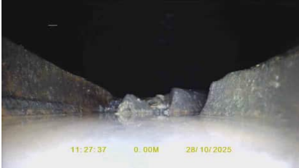
S1X_0a31ed20-f51a-42e6-b7ab-3c21470abb48_20251105_145450_982.jpg, 00:00:00, 0.00 m Start node, inspection chamber, reference: SW1
