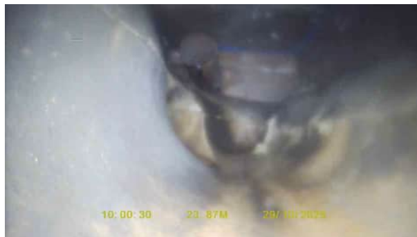
SW8X_7c8a03f6-9105-4766-9955-cb7ec52c0436_20251120_112205_230.jpg, 00:02:21, 23.90 m Finish node, inspection chamber, reference: SW8
