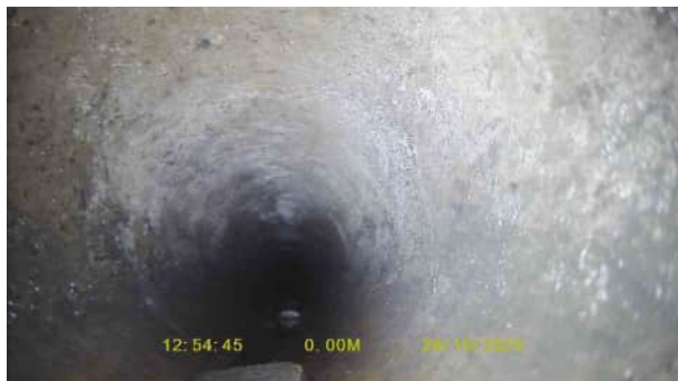
SW4X_a1253e0d-fca4-4160-9ff5-8b137770c5a2_20251105_155228_433.jpg, 00:00:00, 0.00 m Start node, inspection chamber, reference: SW2
