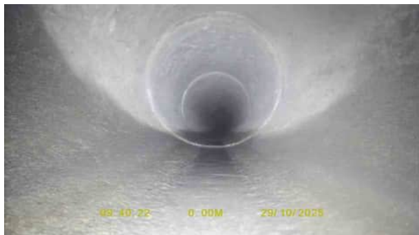
SW6AX_94a35ebe-12e2-4b94-9e8f-4559e47e3013_20251120_104436_067.jpg, 00:00:00, 0.00 m Start node, inspection chamber, reference: SW6
