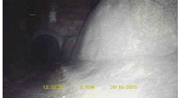
SW3X_170cebc4-96fa-4958-a5b3-038a8b62cad0_20251105_154725_575.jpg, 00:00:24, 2.92 m Finish node, inspection chamber, reference: SW3
