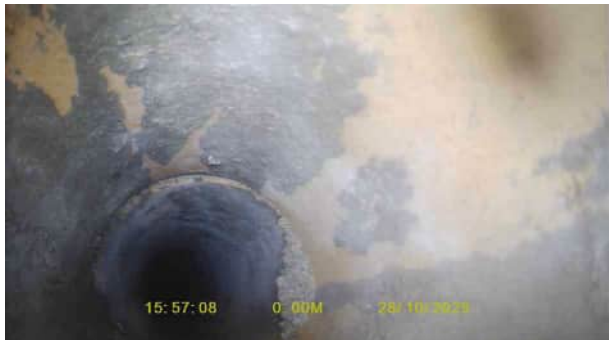
F18X_d12bbb9b-8176-43c7-bce2-37e3255c9796_20251120_095733_616.jpg, 00:00:00, 0.00 m Start node, inspection chamber, reference: FW9
