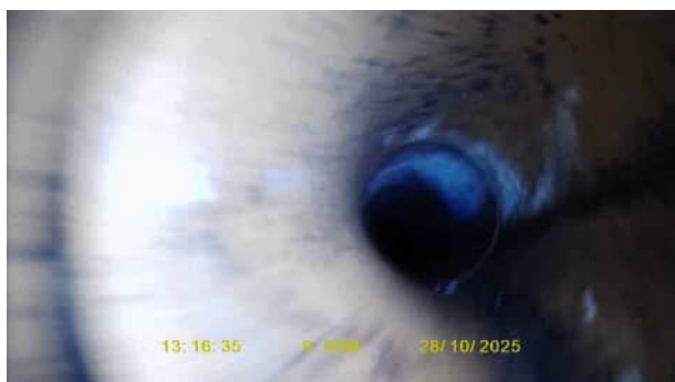
FW4X_77facc1b-5bb4-4911-9460-b696df87e01f_20251111_144013_094.jpg, 00:00:02, 0.50 m Joint displaced, medium
