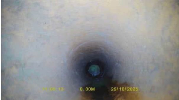
SW9X_41089538-2c0e-4e9a-a427-1a1fc957ec04_20251120_125905_155.jpg, 00:00:00, 0.00 m Start node, inspection chamber, reference: SW8
