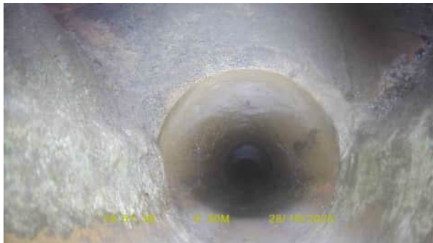
FW9X_1d80b47b-9ebb-4193-960b-379990867af4_20251120_095423_985.jpg, 00:00:00, 0.00 m Start node, inspection chamber, reference: FW8
