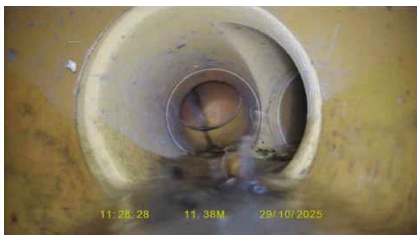
S22X_921f4fa8-1230-4a5f-9aaf-9a18440b6877_20251120_132239_318.jpg, 00:00:52, 11.60 m Junction at 3 o'clock, 100mm dia
