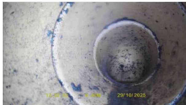
S25X_aac4ad21-e1b7-475c-8e7e-0500be7e5208_20251120_140910_264.jpg, 00:00:48, 9.60 m Finish node, other special chamber, reference: S25, RWP
