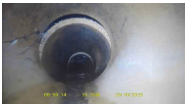
SW8X_4de8e657-5545-49fc-8a57-f15be91d021d_20251120_112035_248.jpg, 00:01:05, 14.15 m Junction at 3 o'clock, 100mm dia
