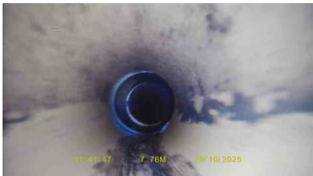
F27X_090e1ad3-ee09-45a2-8c13-56851b860ee8_20251120_133325_419.jpg, 00:00:28, 8.10 m Junction at 9 o'clock, 100mm dia
