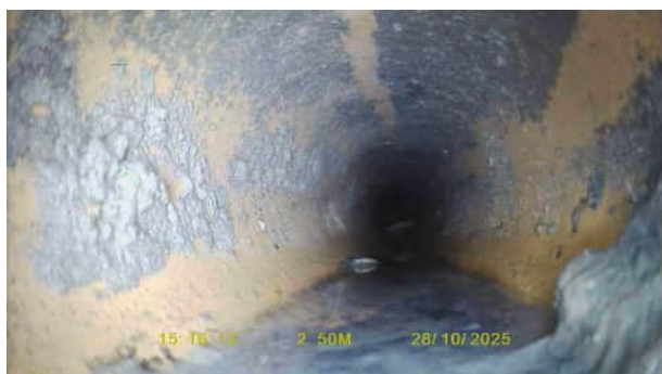
F12X_fb06563c-58f2-4a4c-a0e7-9ae1542b9ff6_20251120_085035_502.jpg, 00:00:36, 2.50 m Survey abandoned, Silt
