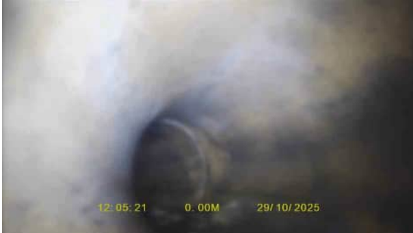
SW13X_3f0dc33b-5fa1-40d5-a62c-03903d441987_20251120_140333_813.jpg, 00:00:00, 0.00 m Start node, inspection chamber, reference: SW11
