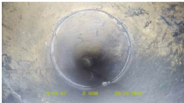
SW7X_c3117112-ce26-44eb-a9a9-9499ff4f2f62_20251112_1 32555_864.jpg, 00:00:00, 0.00 m Start node, inspection chamber, reference: SW3
