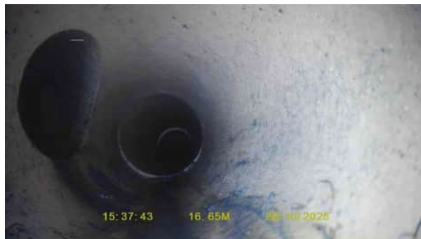
SW12X_3df444a8-75e0-4842-b82c-ee14bf831cbe_20251120_093200_235.jpg, 00:01:16, 16.90 m Junction at 10 o'clock, 100mm dia
