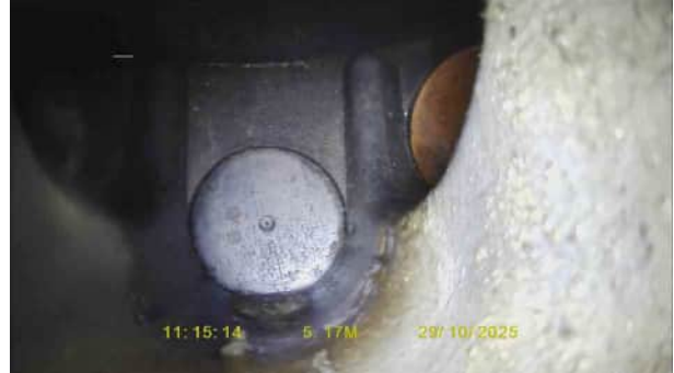
SW10X_8822fee7-2041-4ffc-b841-626dbc3c4355_20251120_131135_160.jpg, 00:00:26, 5.20 m Finish node, inspection chamber, reference: SW10
