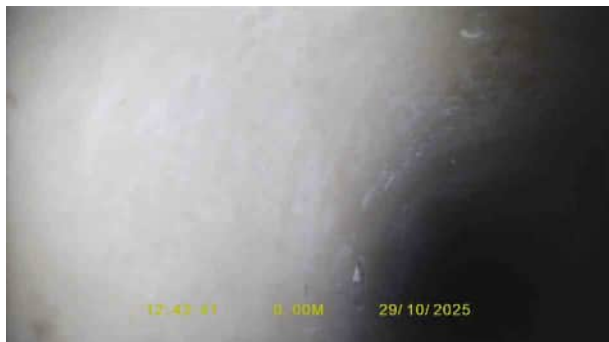
S27X_380cfb4e-3cee-45fe-aa87-0a32545695f6_20251120_1 41609_817.jpg, 00:00:00, 0.00 m Start node, inspection chamber, reference: SW13
