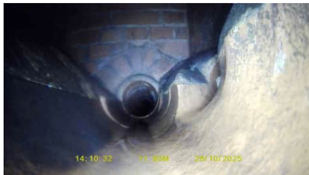
SW7X_35323b36-64ec-4426-a42f-338b75261169_20251112_153424_420.jpg, 00:00:52, 12.00 m Finish node, inspection chamber, reference: SW7
