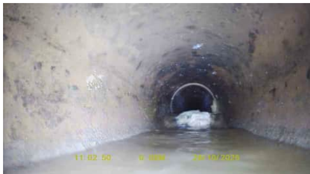
F1X_29c03f47-5be3-4816-8b6e-67b3aa7c93f7_20251105_134808_147.jpg, 00:00:00, 0.00 m Start node, inspection chamber, reference: FW1
