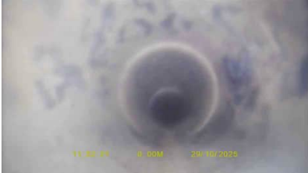
F28X_bb191c79-a988-4738-b69f-8a408ab3b77d_20251120_133952_183.jpg, 00:00:00, 0.00 m Start node, inspection chamber, reference: FW14
