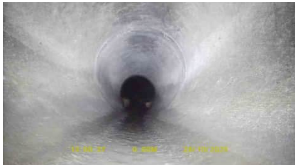
SW2X_a3a8e977-5184-417f-b0ca-f8e21f3dd32b_20251111_142527_486.jpg, 00:00:00, 0.00 m Start node, inspection chamber, reference: SW2
