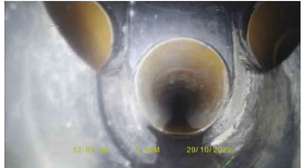
S23X_aeaca6d0-b4e6-4cb8-9f05-7b852b92e00d_20251120_135557_587.jpg, 00:00:39, 5.43 m Finish node, inspection chamber, reference: SW11A
