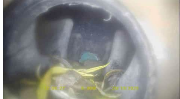
SW13X_099d42ac-5e49-4b4f-84a1-b5c7fd11681f_20251120_140419_078.jpg, 00:01:06, 9.40 m Finish node, inspection chamber, reference: SW13
