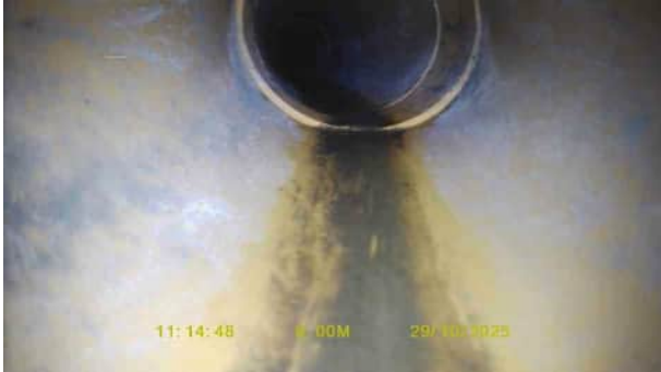
SW10X_2454a701-bbd1-4535-9cba-e00994e87873_20251120_131047_864.jpg, 00:00:00, 0.00 m Start node, inspection chamber, reference: SW11
