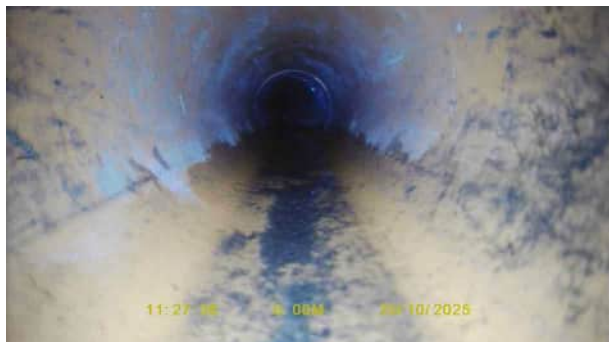
S22X_e935165c-ecee-47df-8288-41a4b179d7fd_20251120_132143_637.jpg, 00:00:00, 0.00 m Start node, inspection chamber, reference: SW9
