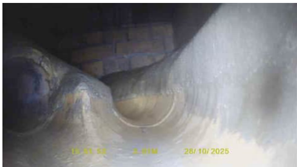
FW9X_299f47fb-1462-41f1-a33b-e55f59191c6a_20251120_095519_806.jpg, 00:00:15, 3.00 m Finish node, inspection chamber, reference: FW9
