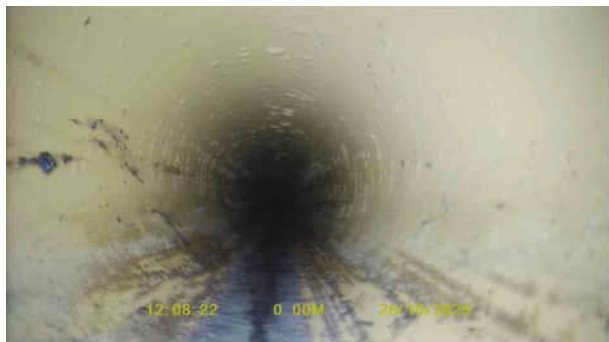
FW2X_5325331a-964a-45fd-8d86-de063a378b84_20251105_150300_600.jpg, 00:00:00, 0.00 m Start node, inspection chamber, reference: FW2
