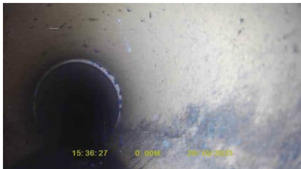
SW12X_6eee9148-6847-487b-a1e0-3181cf1758f7_20251120_092806_124.jpg, 00:00:00, 0.00 m Start node, inspection chamber, reference: SW5
