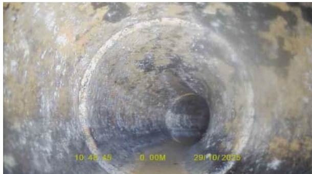
FW12AX_894953b8-0c28-4071-a2ac-eb830aa5e765_20251120_123944_093.jpg, 00:00:00, 0.00 m Start node, inspection chamber, reference: FW12
