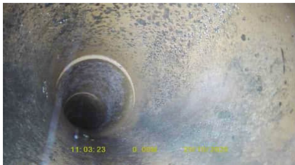
S17X_3fff4aaa-7bbd-428e-95b4-7b3ae694cc70_20251120_1 25058_619.jpg, 00:00:00, 0.00 m Start node, inspection chamber, reference: SW8
