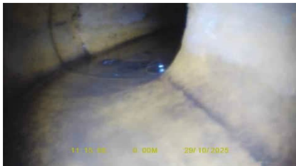
S21X_e9b26a55-3493-4c42-a1f7-e1afb6c1fdca_20251120_13 1507_759.jpg, 00:00:00, 0.00 m Start node, inspection chamber, reference: SW9
