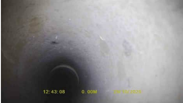
S26X_db73b9a0-2c9b-48f3-8806-0531617e4b8a_20251120_141246_805.jpg, 00:00:00, 0.00 m Start node, inspection chamber, reference: SW13
