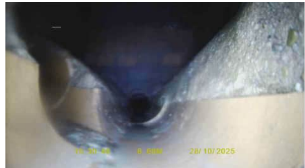
FW8X_c4952df1-13be-438a-9fc4-9c86633f050b_20251120_091445_153.jpg, 00:00:27, 6.70 m Finish node, inspection chamber, reference: FW8
