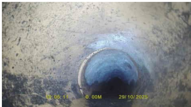
S15X_9fd4bcaa-79a4-4037-b7f6-ca040c1902e6_20251120_1 12744_318.jpg, 00:00:00, 0.00 m Start node, inspection chamber, reference: SW7
