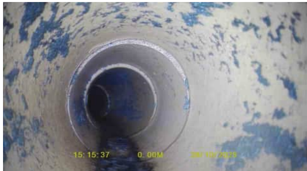
F12X_4af88f0c-0f7e-429b-94e7-21a77dd8652d_20251120_084914_757.jpg, 00:00:00, 0.00 m Start node, inspection chamber, reference: FW5
