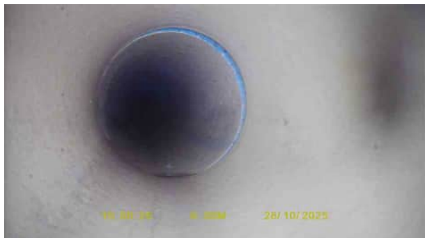
F16X_3dec09ef-61b2-4e63-b174-4c457b96bb01_20251120_094631_178.jpg, 00:00:00, 0.00 m Start node, inspection chamber, reference: FW8
