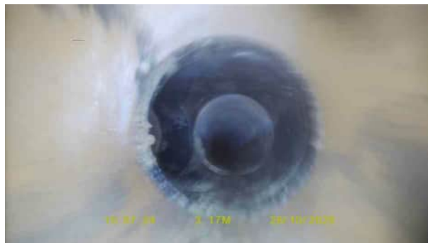
F18X_90043daa-d39f-433c-adae-6718dd3bdc0d_20251120_095852_397.jpg, 00:00:17, 3.20 m Junction at 9 o'clock, 100mm dia
