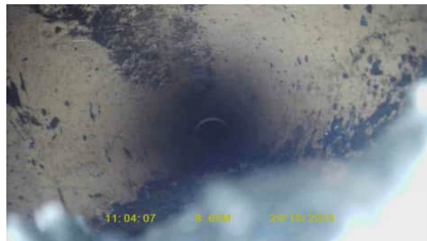
S17X_334b8896-3de8-4452-9fb8-f5e9f4b0ef82_20251120_12 5152_380.jpg, 00:00:45, 8.65 m Survey abandoned, Silt
