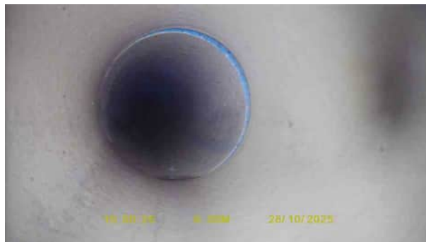
F16X_0a61345b-0ac1-41b1-8dbf-4b5e32534f95_20251120_094648_141.jpg, 00:00:00, 0.10 m Joint displaced, medium
