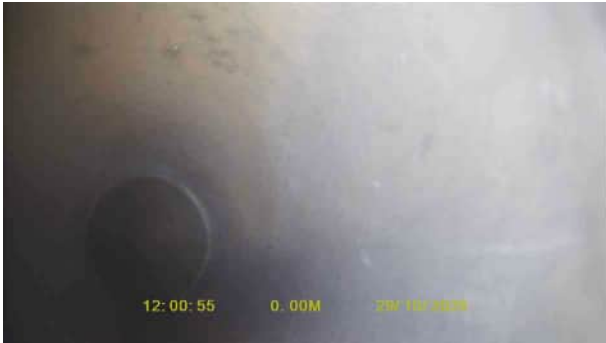
S23X_40c6d6b5-380d-412b-9961-6e55b0c174ac_20251120_135201_332.jpg, 00:00:00, 0.00 m Start node, inspection chamber, reference: SW11
