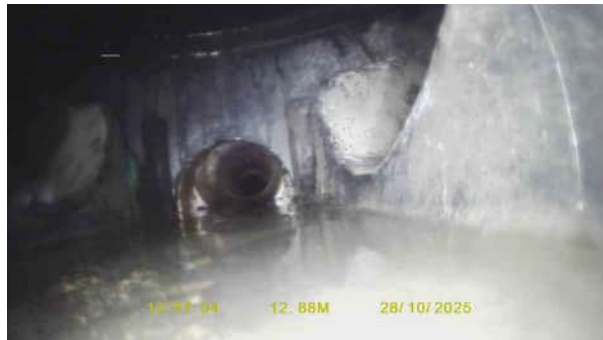
SW4X_58c1287e-d734-4c0e-ab6d-237c6487005a_20251105_161810_084.jpg, 00:02:20, 12.90 m Finish node, inspection chamber, reference: SW4
