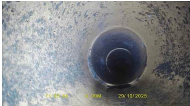
SW11X_a03ef129-6c9d-46c4-8a55-0b6fa993e1df_20251120_130225_394.jpg, 00:00:00, 0.00 m Start node, inspection chamber, reference: SW8
