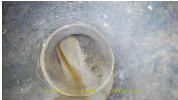
F29X_c6789ac2-5bf9-43df-aa9f-c744bd57e938_20251120_14 2254_962.jpg, 00:00:14, 2.10 m Finish node, other special chamber, reference: F29, WP
