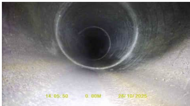
SW6X_53792017-383f-4ada-a9e6-d599aa3ae927_20251112_125503_317.jpg, 00:00:00, 0.00 m Start node, inspection chamber, reference: SW3
