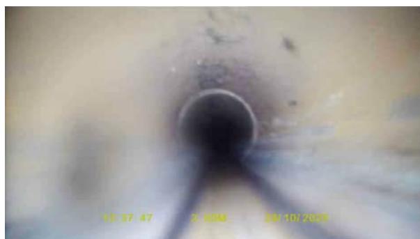
FW3X_e6bc3317-0dc7-4658-ab6d-99b905ed7266_20251112_113822_607.jpg, 00:00:08, 2.60 m Settled deposits, fine, 5% cross-sectional area loss, finish
