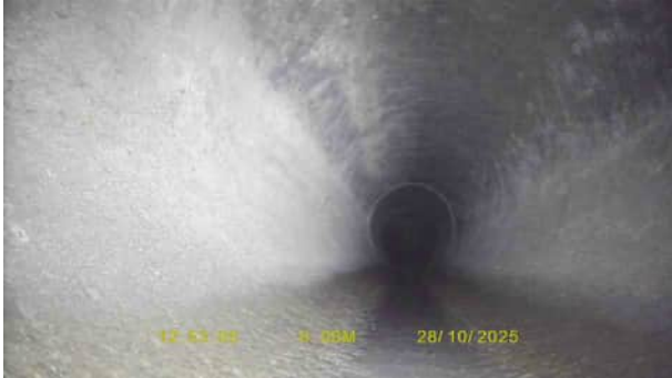
SW3X_a05e0fac-11ce-42d6-b2db-f76f16eb24ed_20251105_154402_714.jpg, 00:00:00, 0.00 m Start node, inspection chamber, reference: SW2
