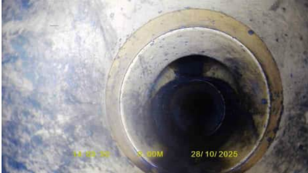
S4X_b22073b4-2a84-4581-9a4e-1c72273a0279_20251112_1 20838_281.jpg, 00:00:00, 0.00 m Start node, inspection chamber, reference: SW3
