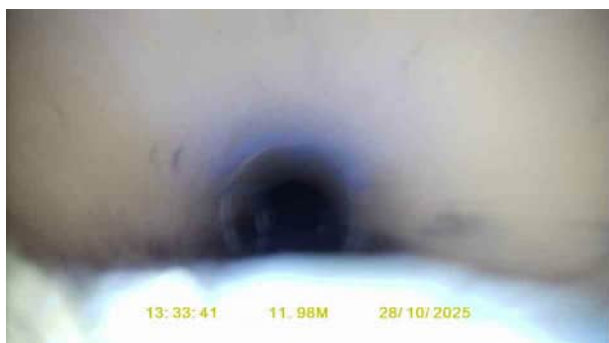
FW5X_d4d2ce8c-e55e-44de-b628-a2b478a5d3fd_20251112_105053_872.jpg, 00:00:46, 12.10 m Joint displaced, medium
