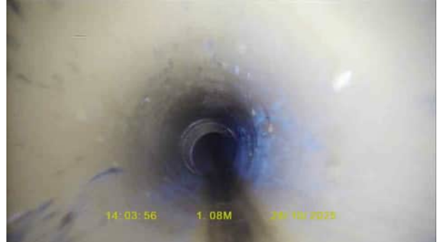
S4X_6d5067f4-d3fd-4022-8af4-fcdee841e3e4_20251112_121 053_909.jpg, 00:00:07, 1.70 m Line deviates up
