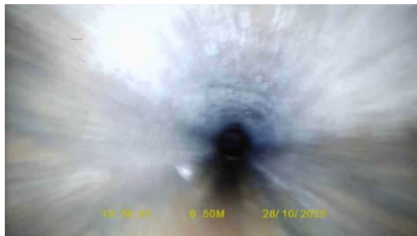
FW10X_20bd3924-e9d3-4552-9ea4-787c0de0be64_20251112_092212_407.jpg, 00:00:05, 1.40 m Joint displaced, medium
