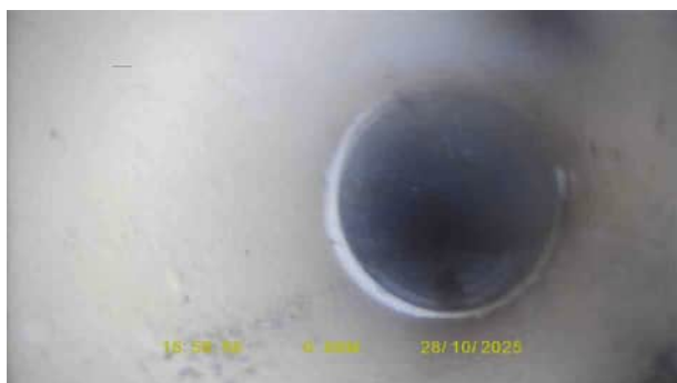
F19X_735fbdf6-34e5-4209-ac70-a1b61ea1732f_20251120_101353_138.jpg, 00:00:05, 1.00 m Joint displaced, medium
