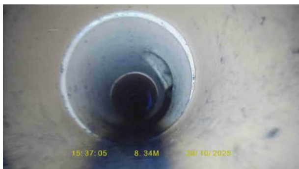
SW12X_fb8a7d7c-65b0-471f-9efa-942eb8d63659_20251120_093051_596.jpg, 00:00:38, 8.80 m Junction at 2 o'clock, 100mm dia
