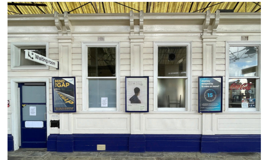
Figure 4.8n: Existing sash windows
