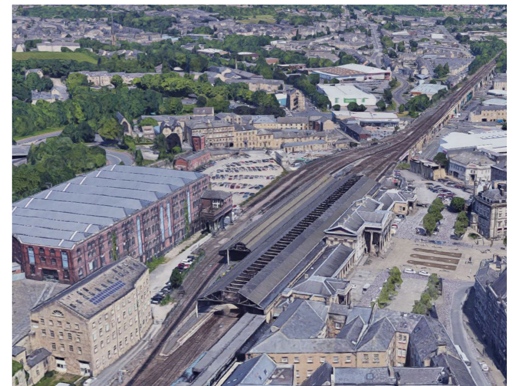
Figure 2.1d: Looking north over Huddersfield viaduct
