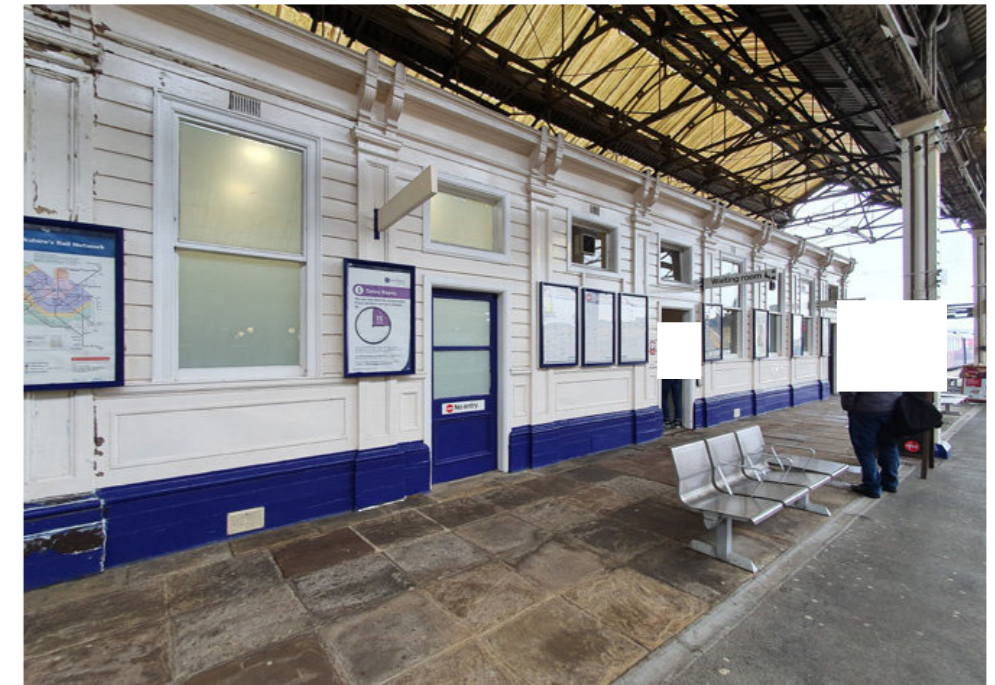
Figure 4.8a: The Tea Rooms prior to dismantling
