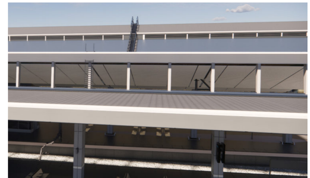
Figure 4.4d: View of clerestory cladding from the LYR warehouse
