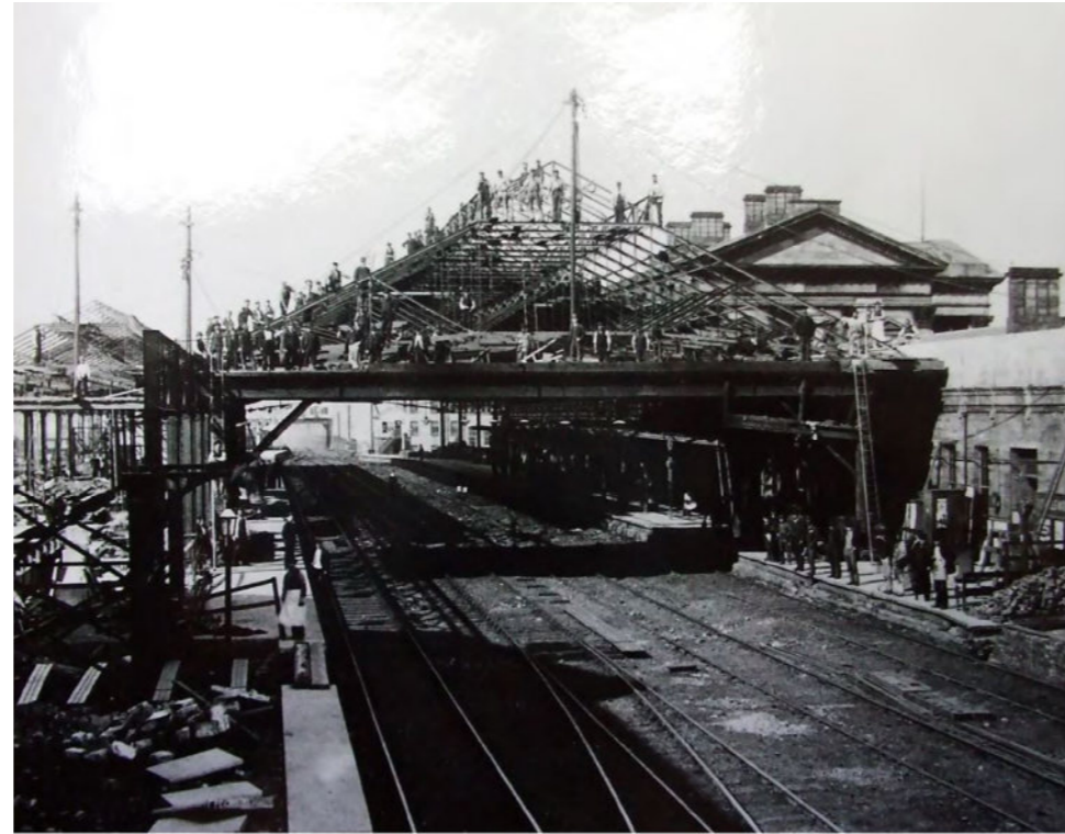
Figure 2.2.3a: Trainsheds under construction 1886
