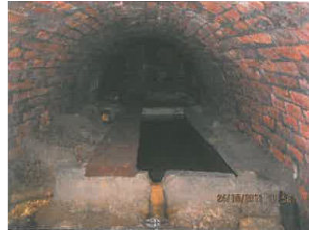
Figure 4.7e: John William Street culvert
