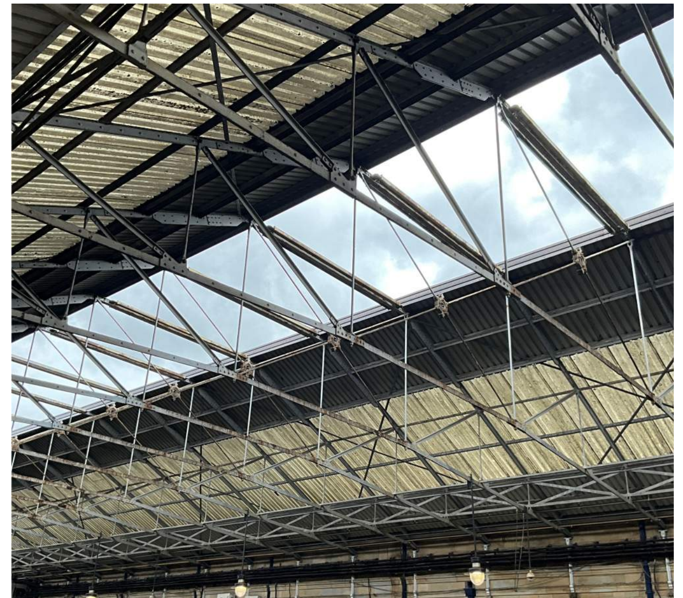
Roof A - Typical Roof A photo from 25.07.2023
