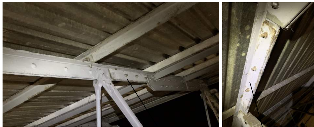
Historic side plate strengthening
