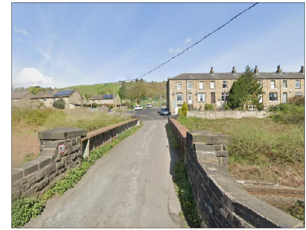
Photo 2 (Looking North West) Scale N.T.S
