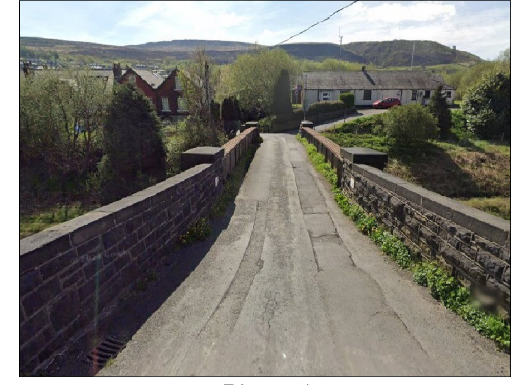
Photo 1 (Looking South East) Scale N.T.S
