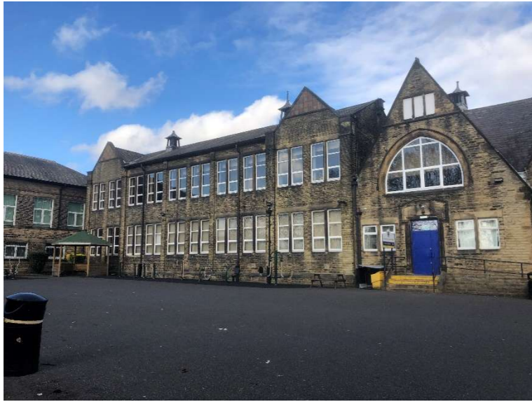
Victorian Stone original Building
