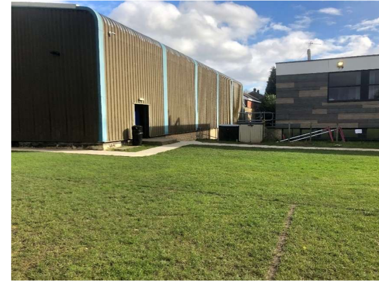
Metal Cladding to Sports Hall late 20 Century
