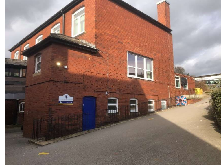
Early 20 century Brick Addition
