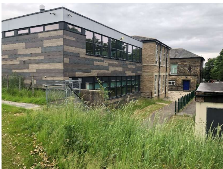
Rainscreen Cladding Modern Refurbishment
