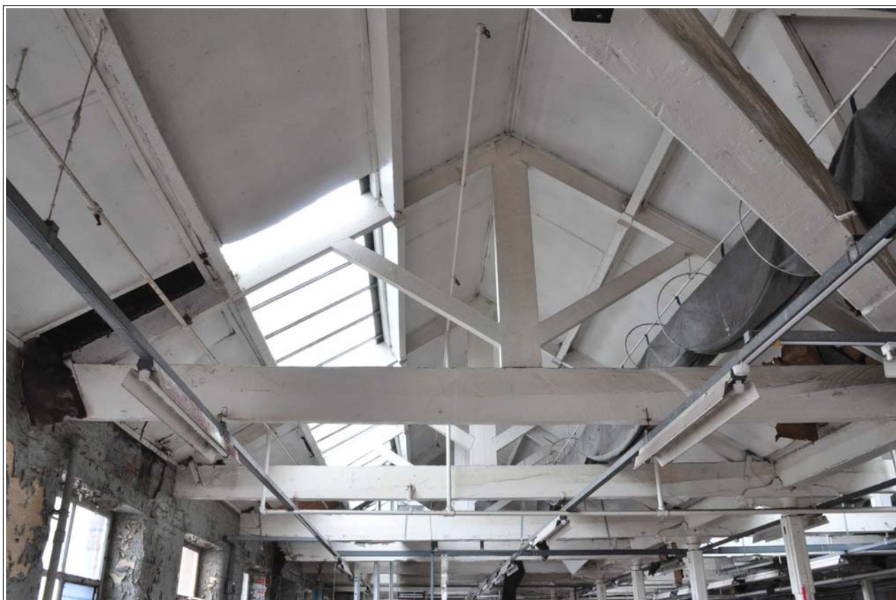
37: Building B (spinning block): roof structure over fifth floor, looking east
