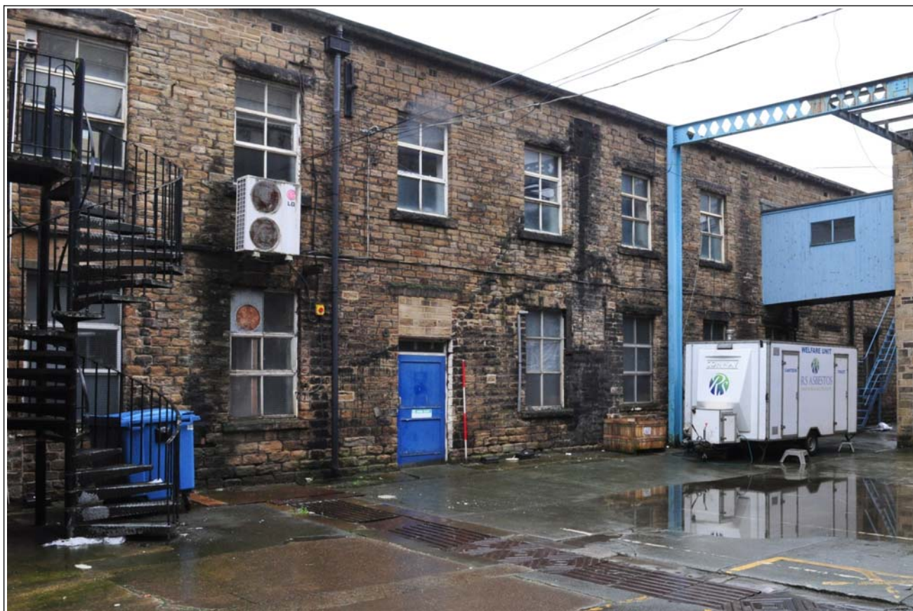
69: Building E (mill/warehouse), looking north-west
