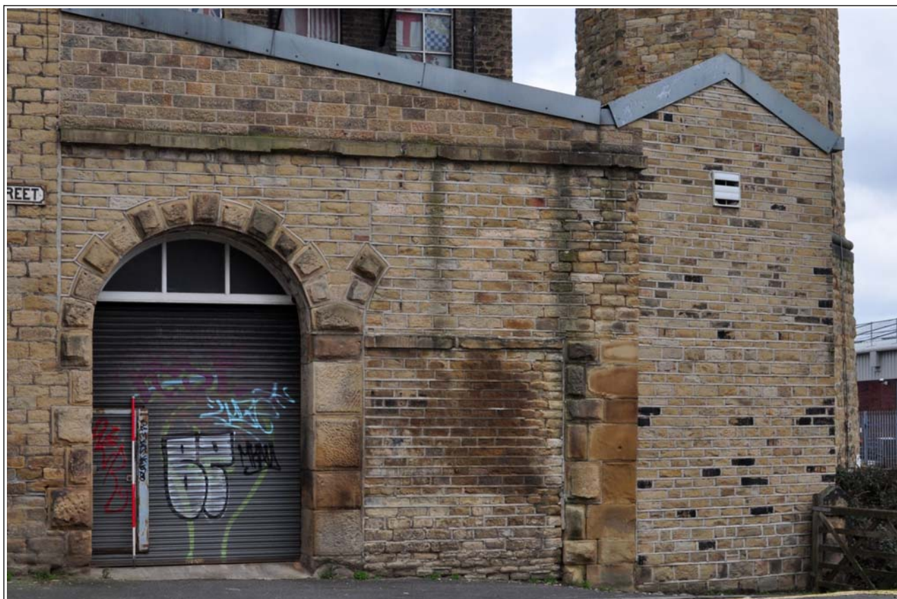
57: Building C (boiler house): south front, with re-built part to right
