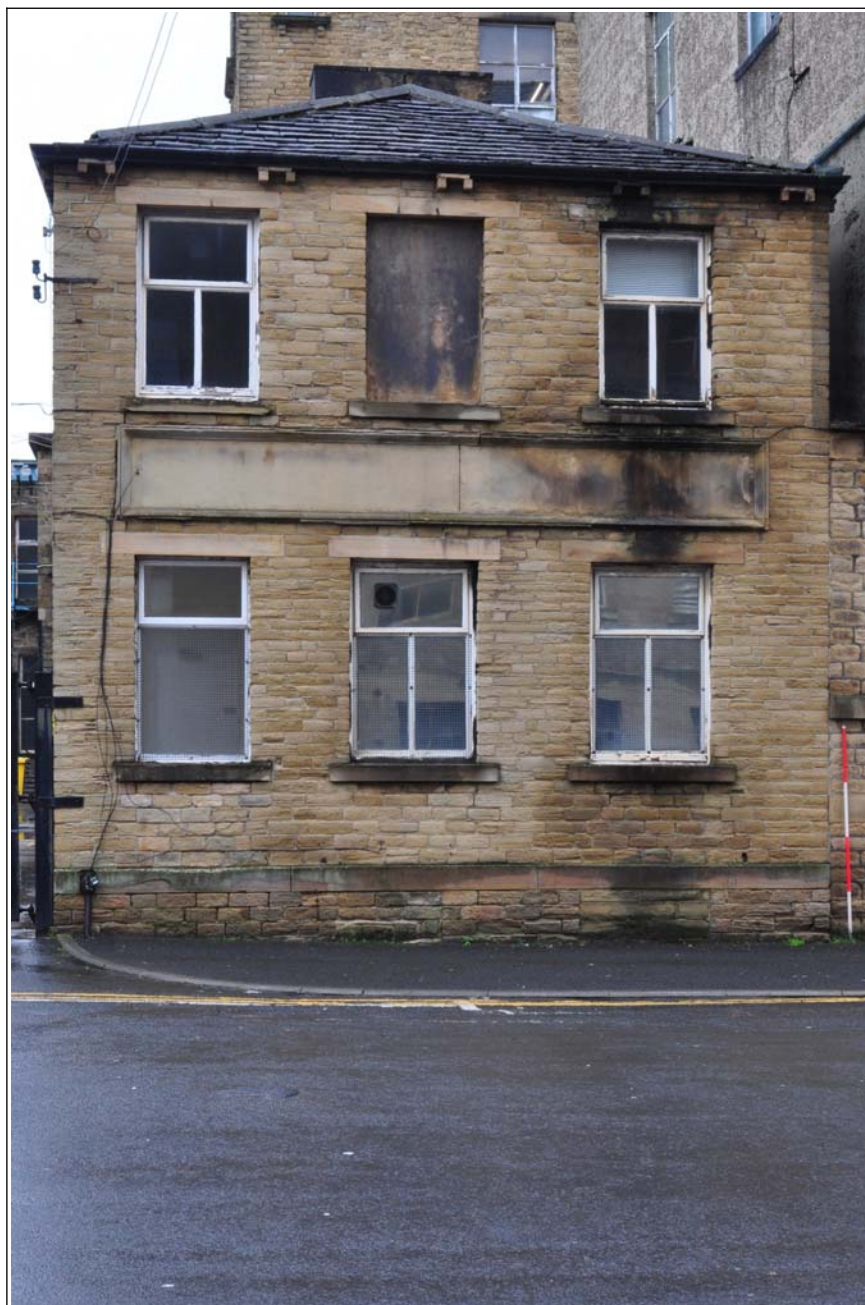
64: Building D1 (offices), south front
