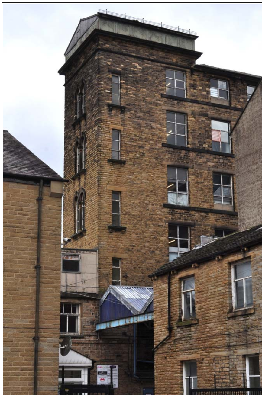
04: Building B (spinning block): stair tower, looking north-east
