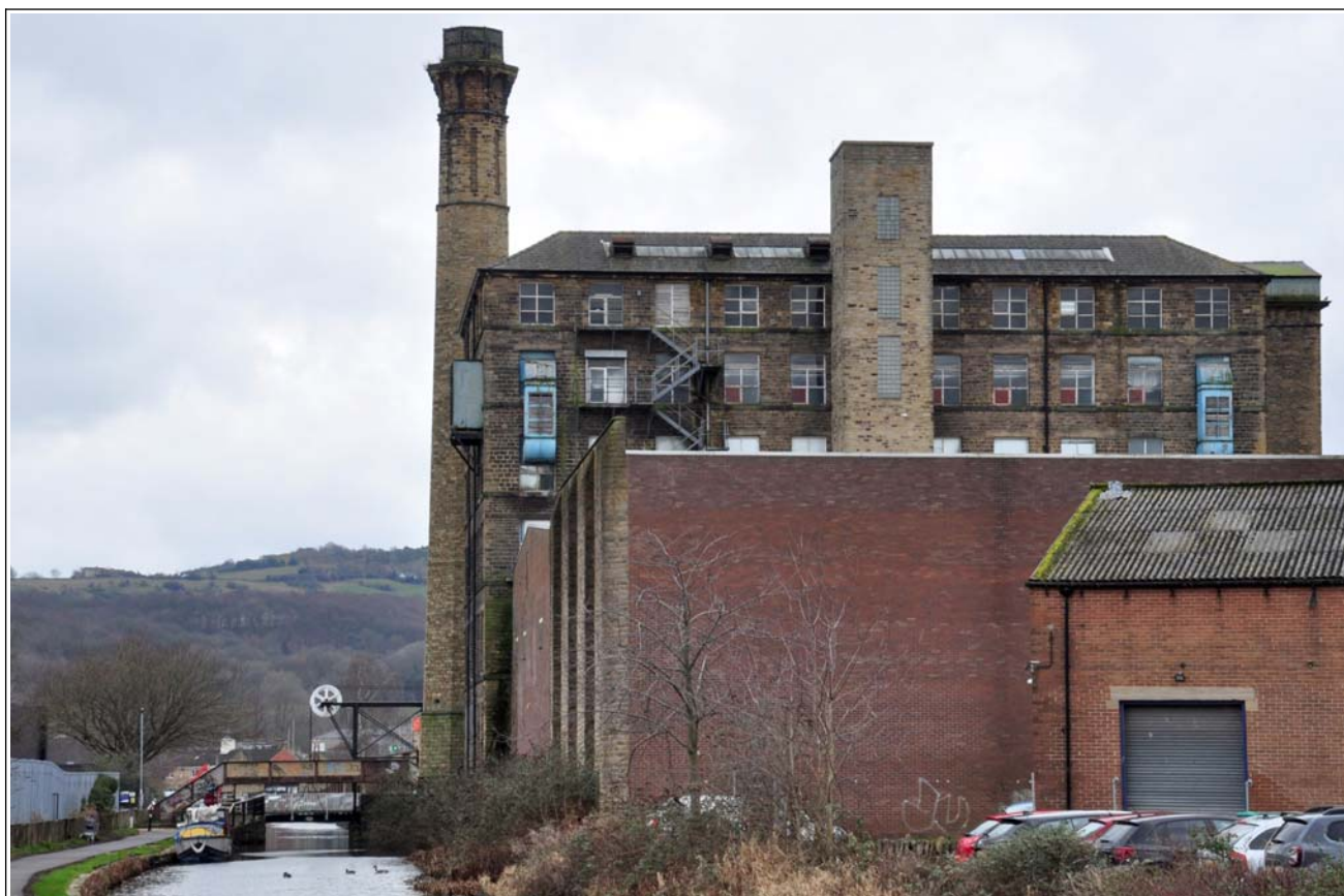
19: Building B (spinning block): general view looking south, across canal
