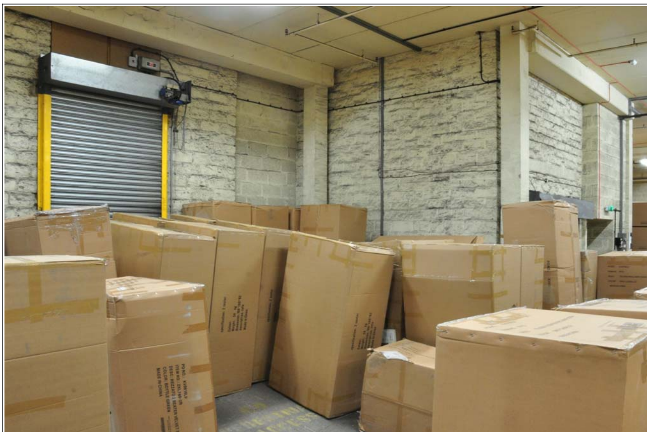
20: Building B (spinning block): part of north elevation with modern lift tower, within modern warehouse
