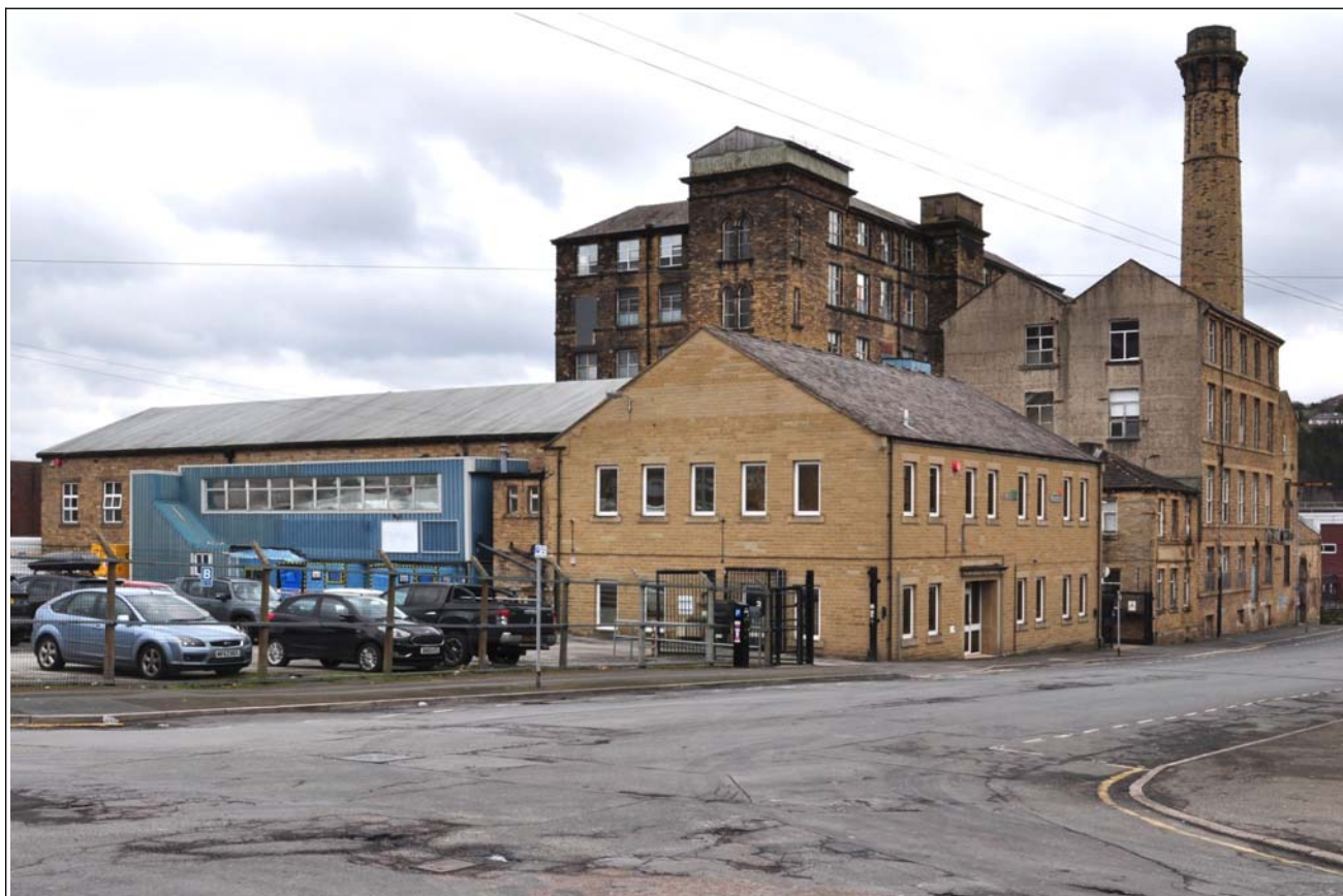
01: General view of the site, looking north-east
