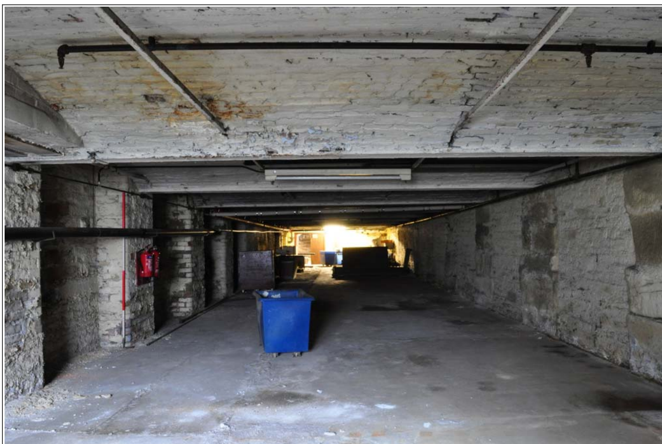
38: Building B (spinning block): basement, looking west
