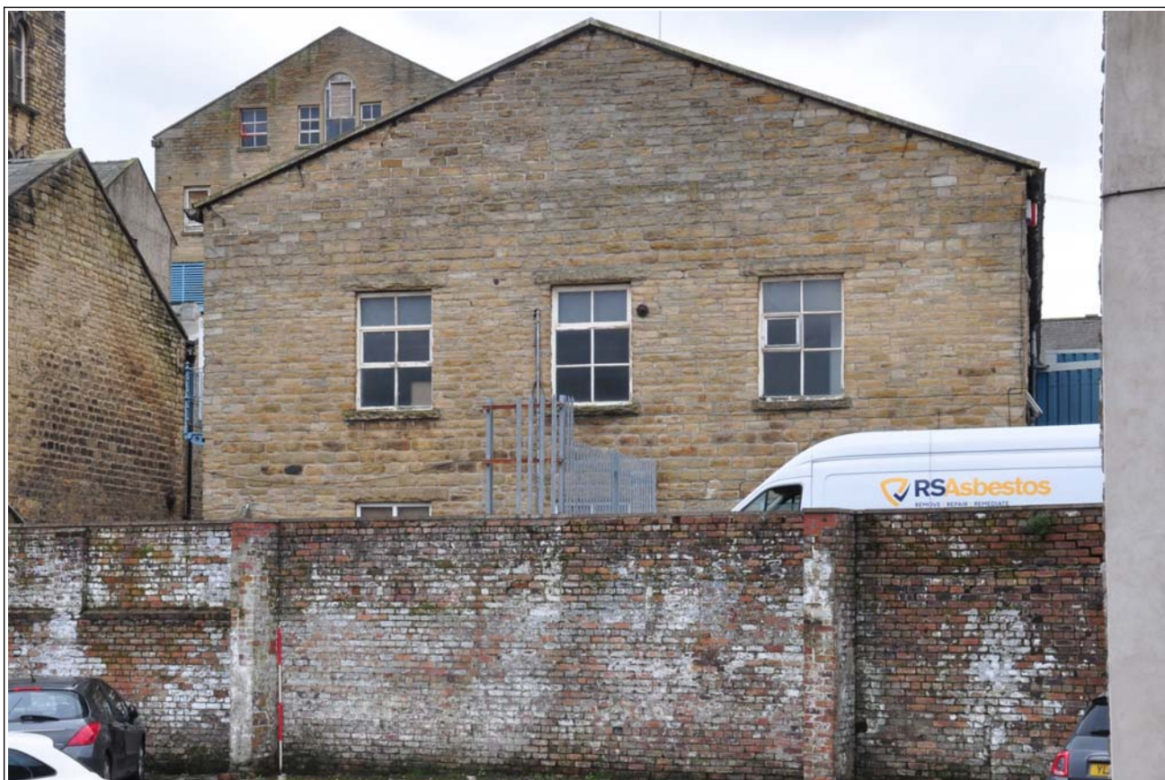
73: Building E (mill/warehouse): north gable
