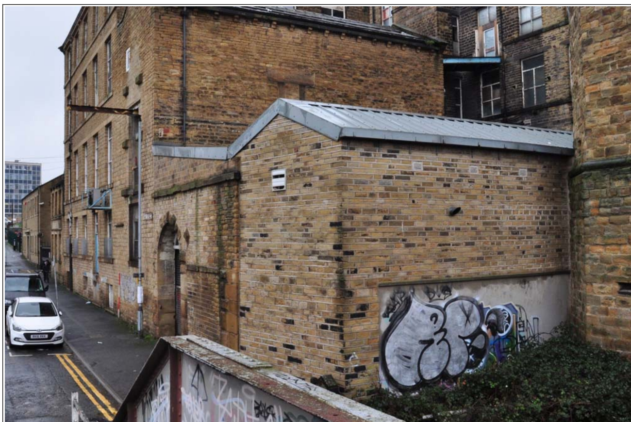
58: Building C (boiler house), looking north-west, with re-built part in foreground
