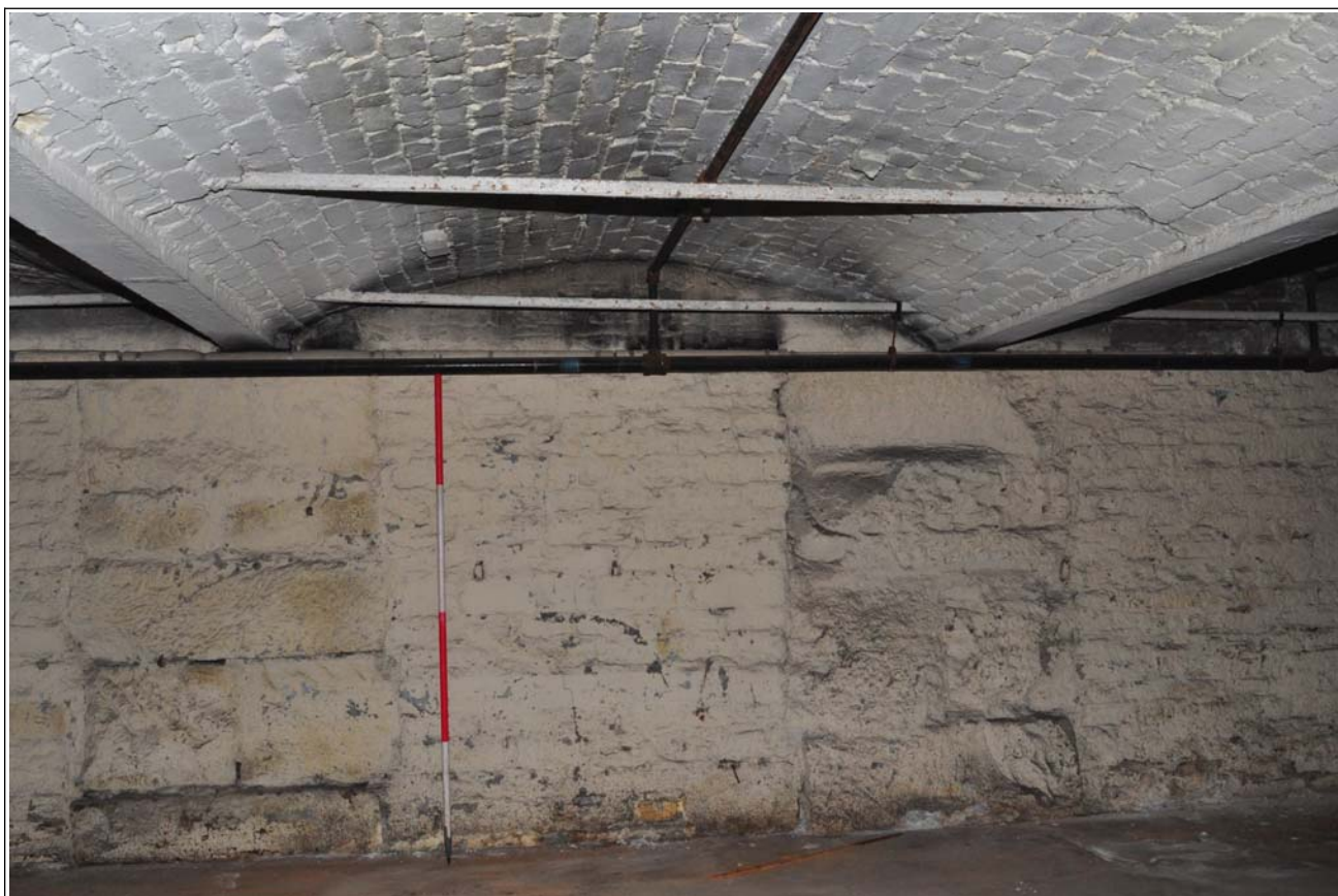
39: Building B (spinning block): north wall of basement
