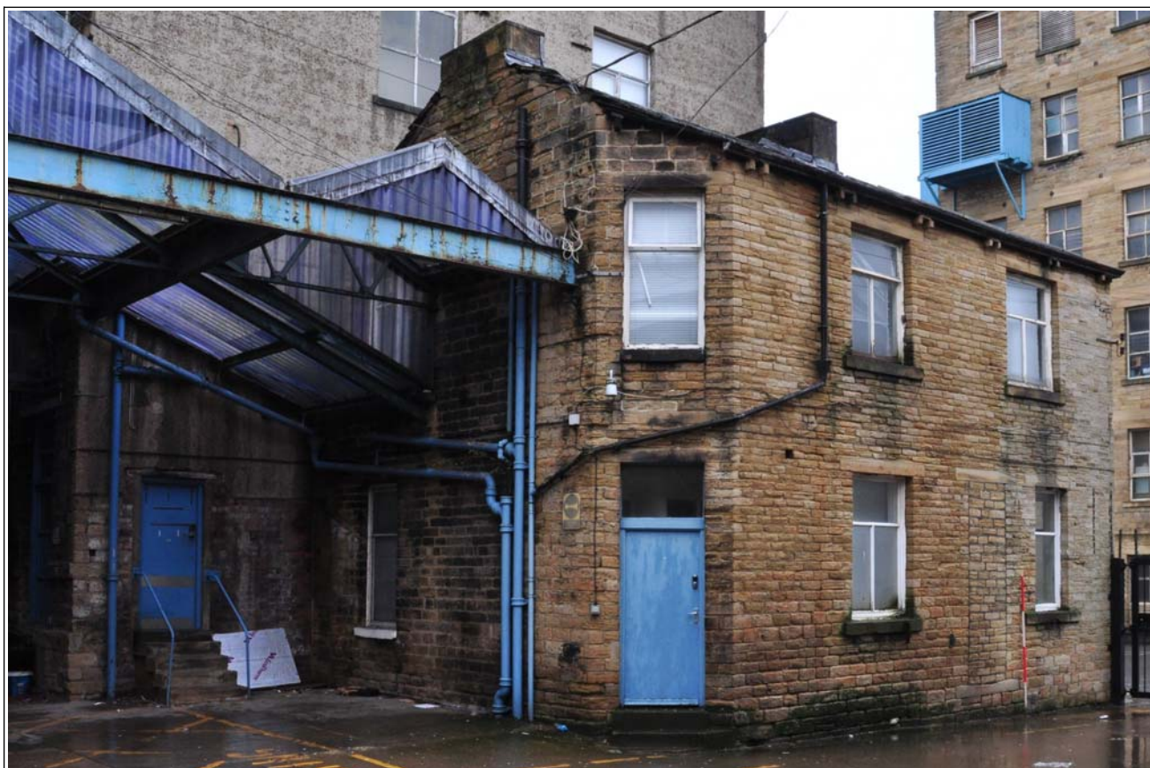
65: Building D1 (offices), looking south-east
