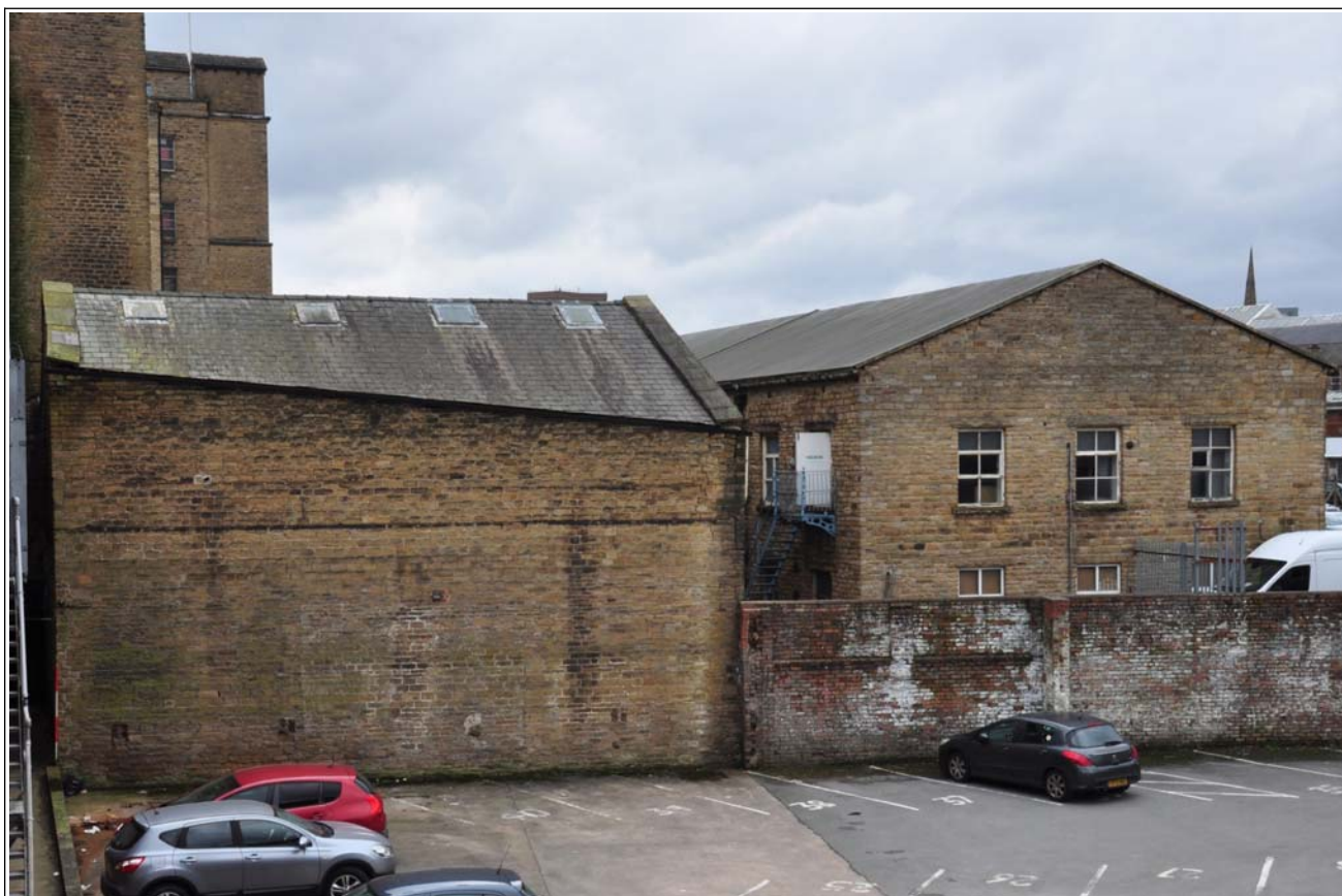
79: Building G (store), looking south towards rear, with building E to right
