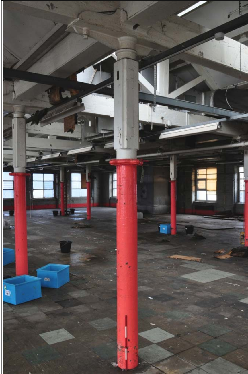
36: Building B (spinning block): typical column on fifth floor, looking south-east
