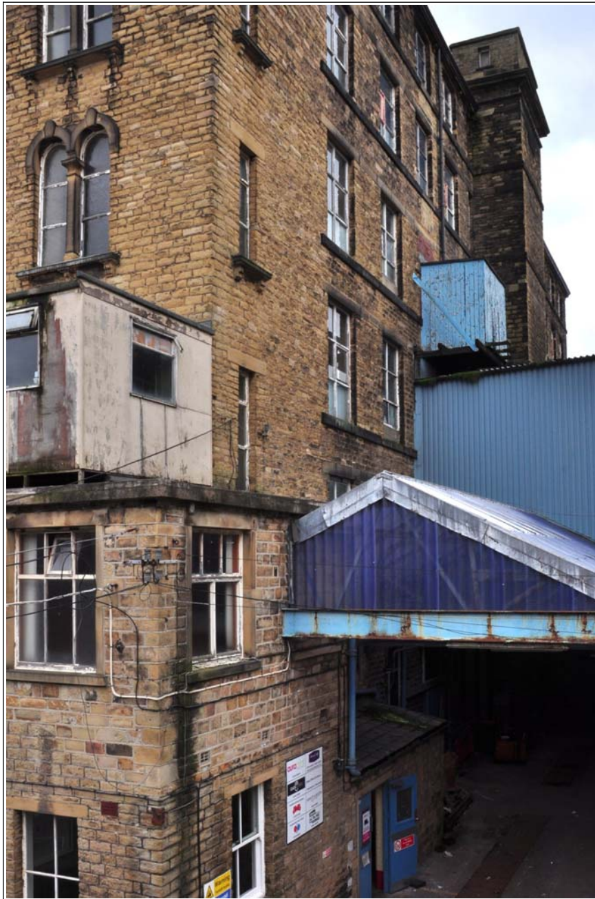
09: Building B (spinning block): upper part of south elevation
