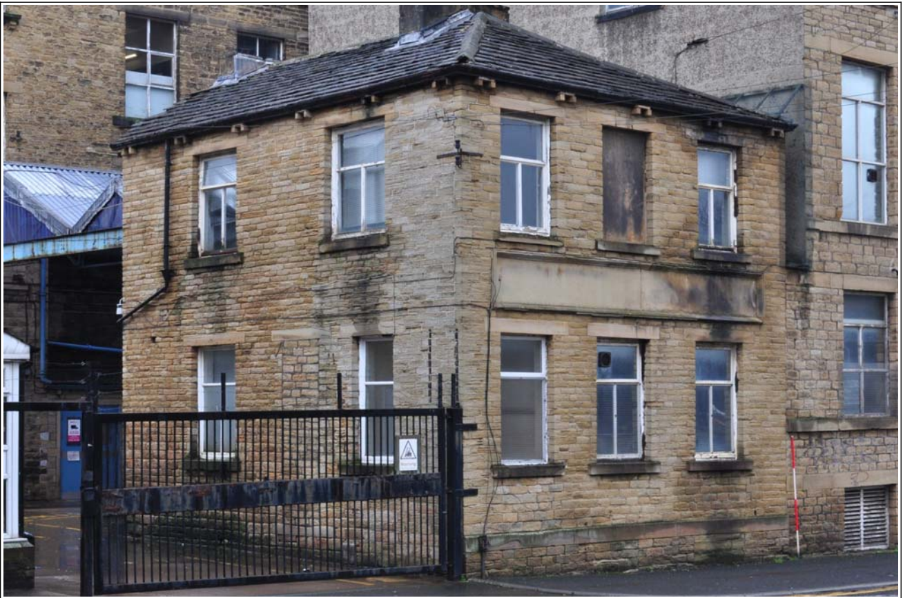
63: Building D1 (offices), looking north-east
