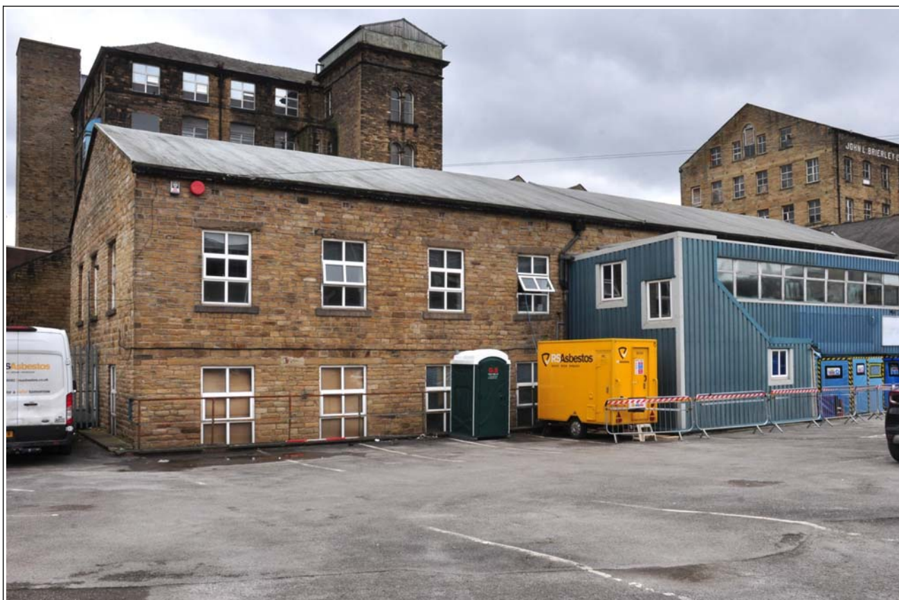
68: Building E (mill/warehouse), looking south-east
