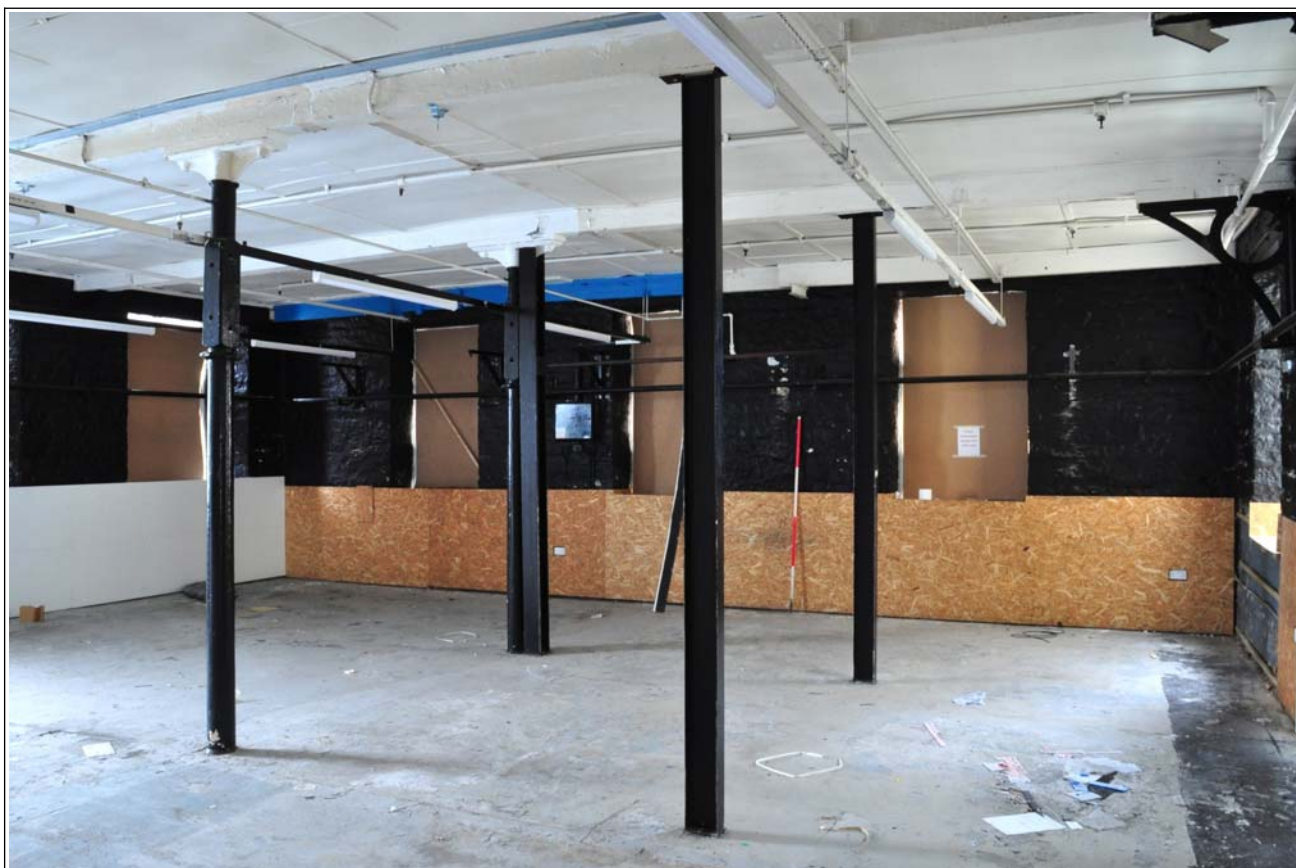
75: Building E (mill/warehouse): ground floor, looking north-west
