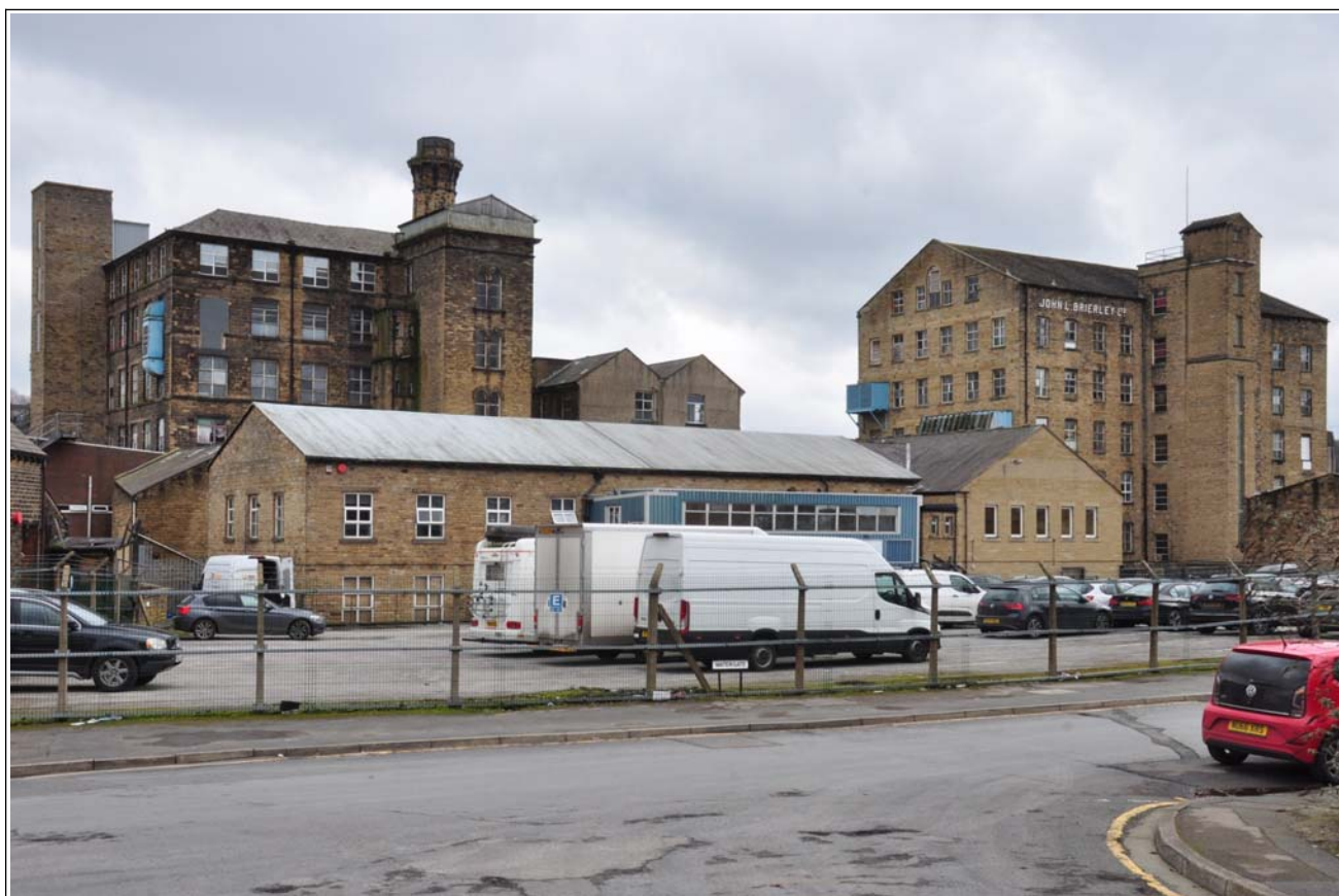
02: General view of the site, looking south-east
