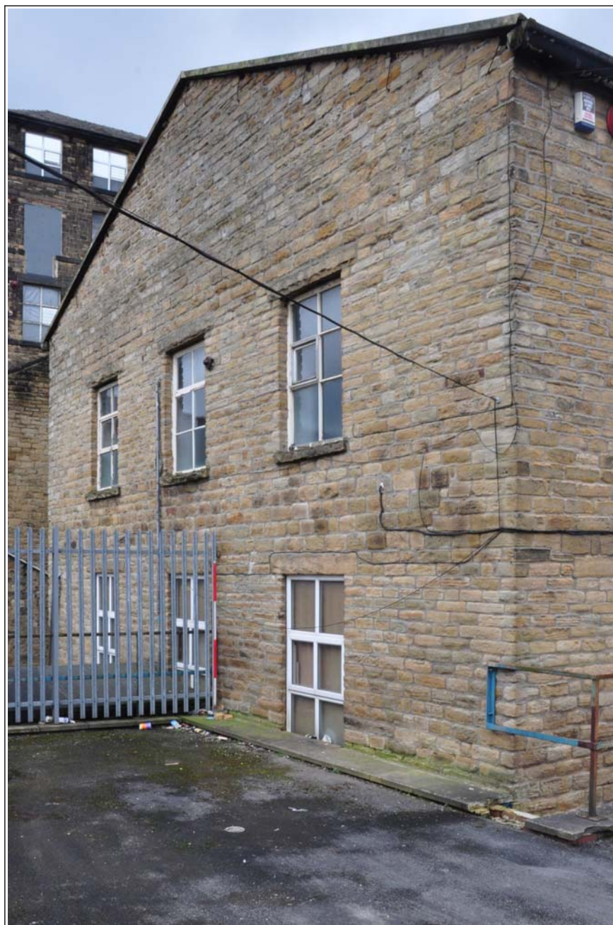
72: Building E (mill/warehouse): north gable
