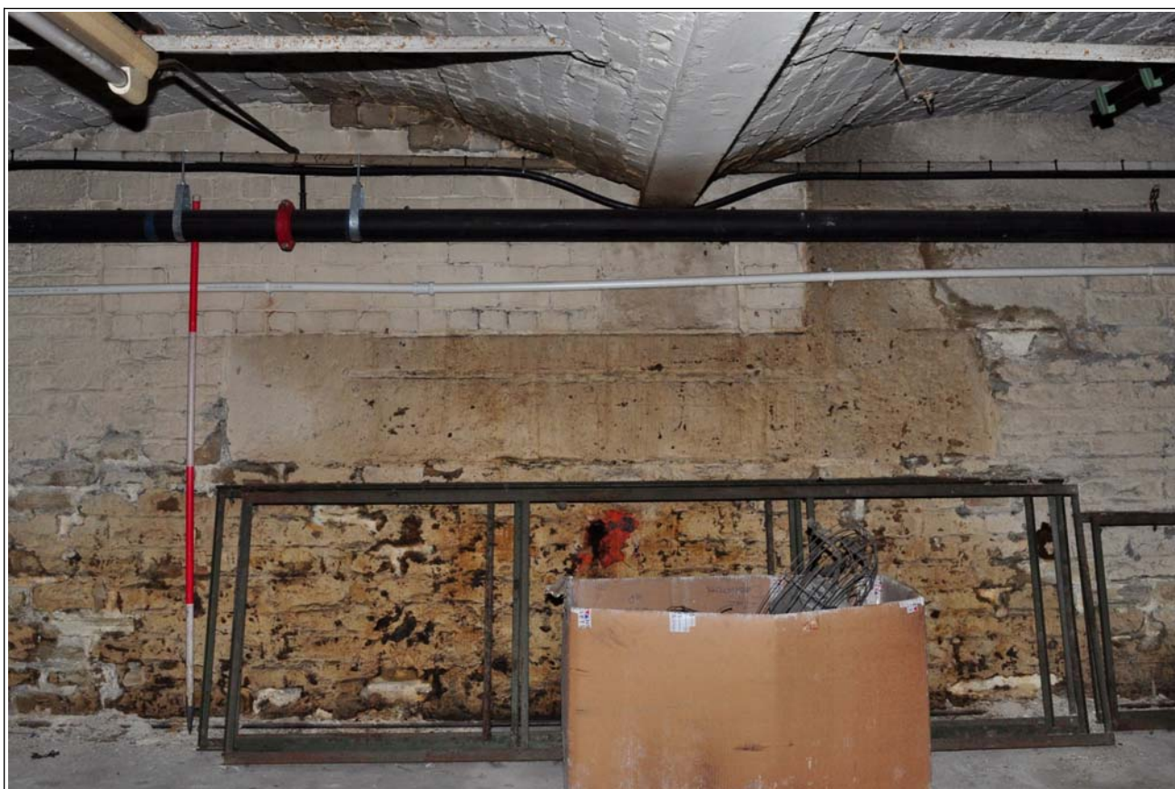
40: Building B (spinning block): south wall of basement, showing massive stone block in line with south shaft/lift tower
