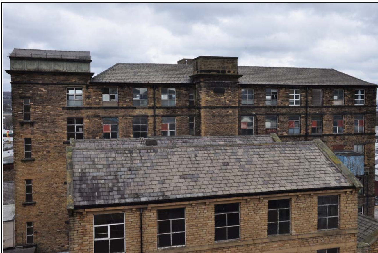
03: Building B (spinning block): upper part of south elevation
