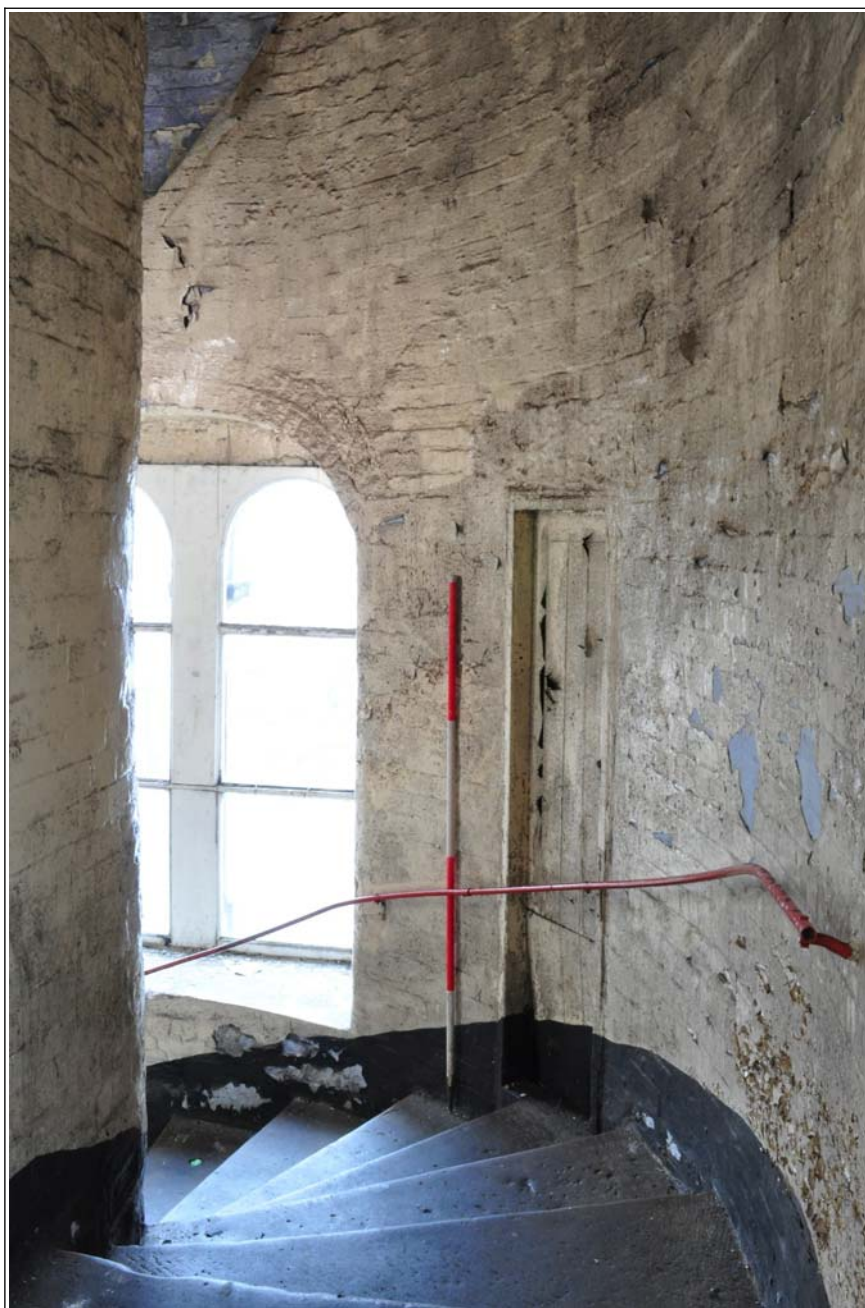
48: Building B (spinning block): stair tower on fifth floor, looking down to the west
