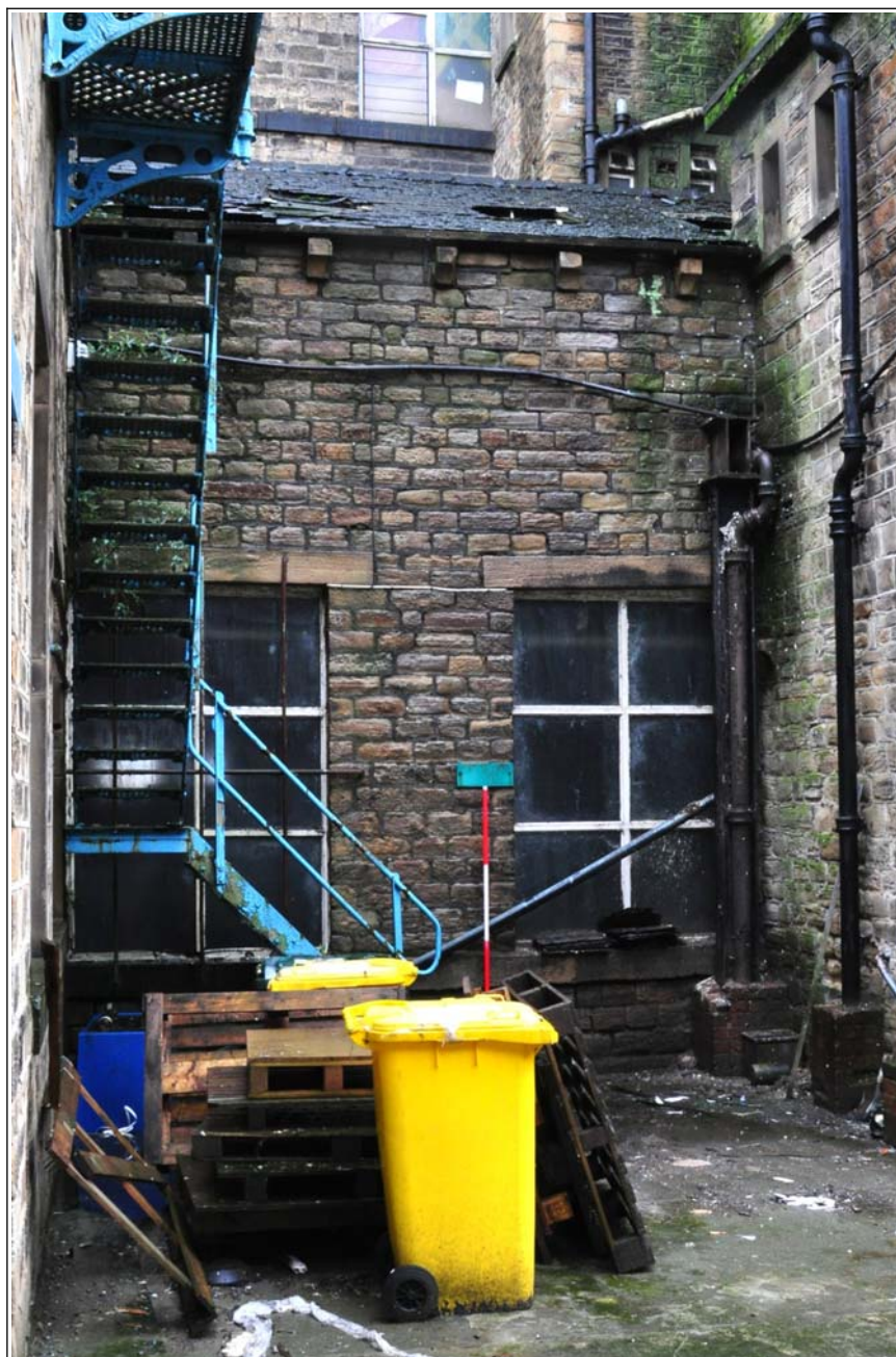
16: Building B (spinning block): extension on west elevation of ca. 1900
