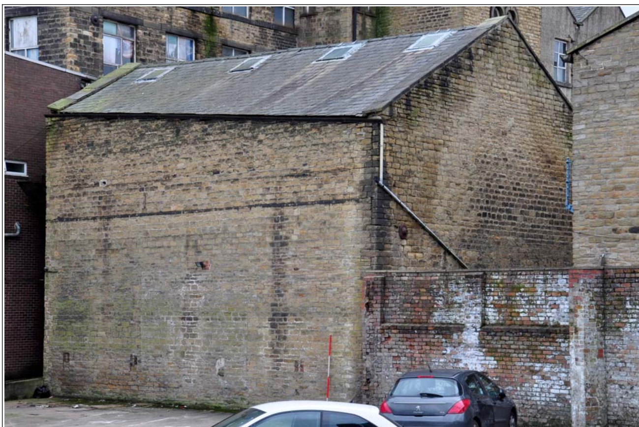
80: Building G (store), looking south-east towards rear
