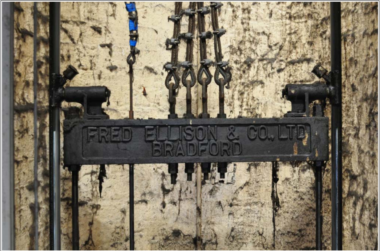
51: Building B (spinning block): stair tower on first floor - name-plate on lift apparatus (20th century)
