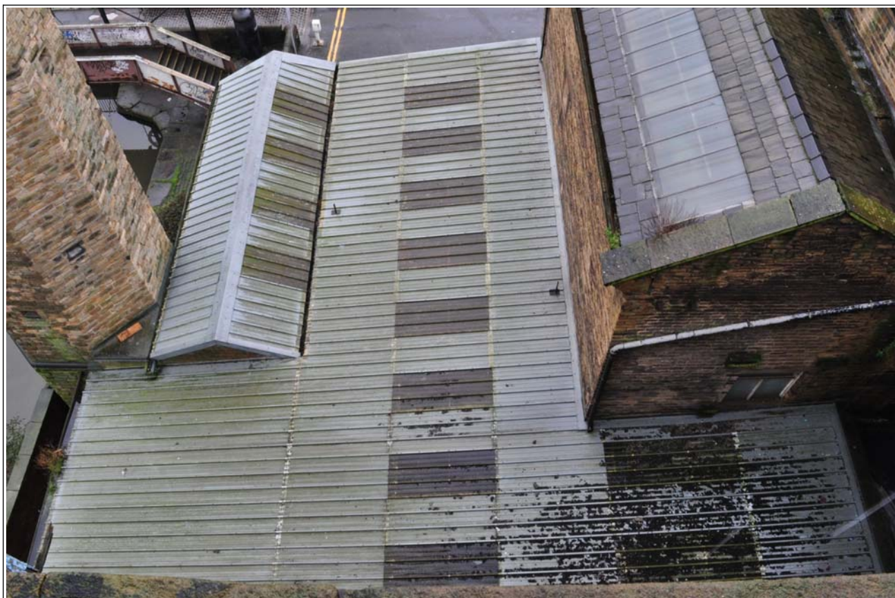
60: Building C (boiler house), looking down onto roof, from the north
