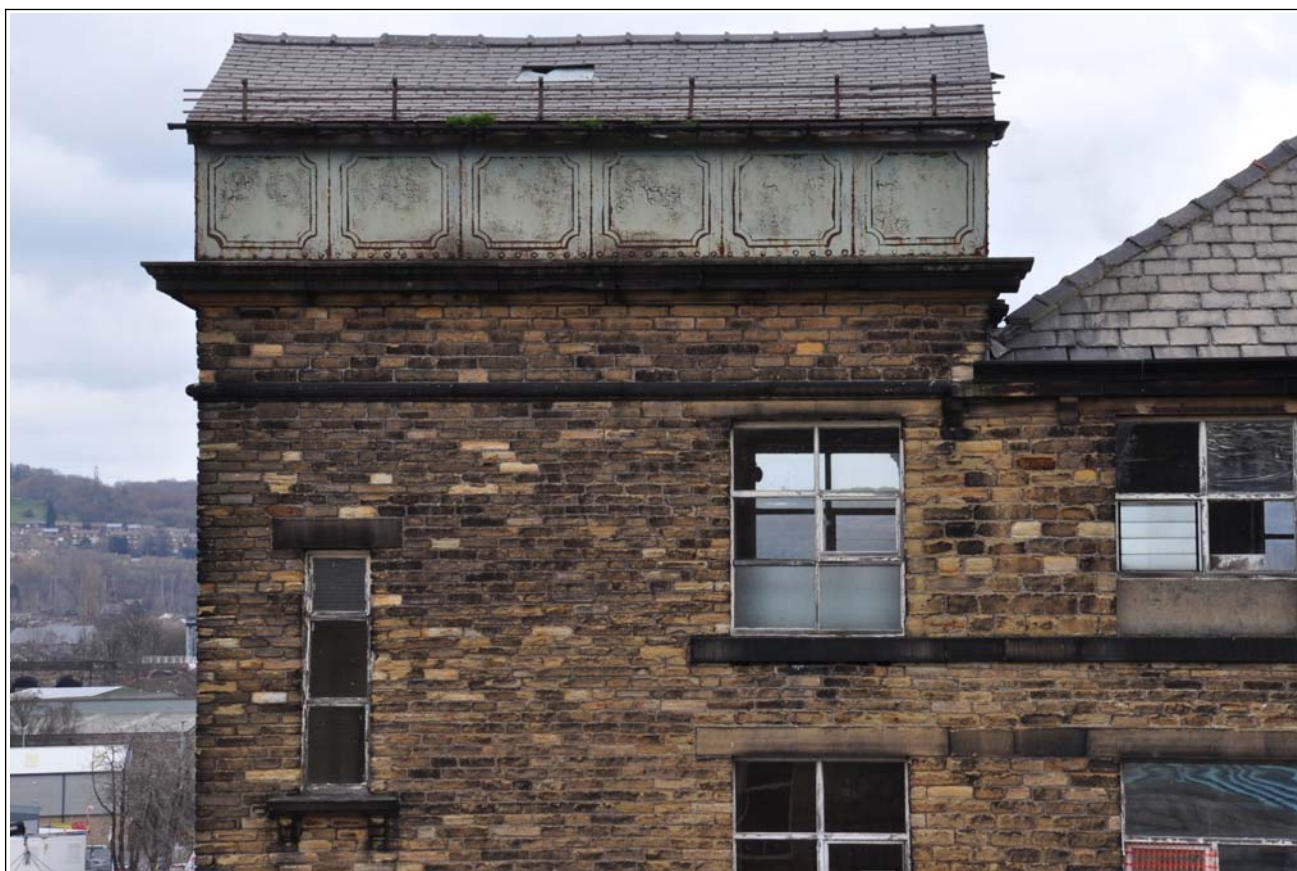
13: Building B (spinning block): water tank and top of stair tower, looking north
