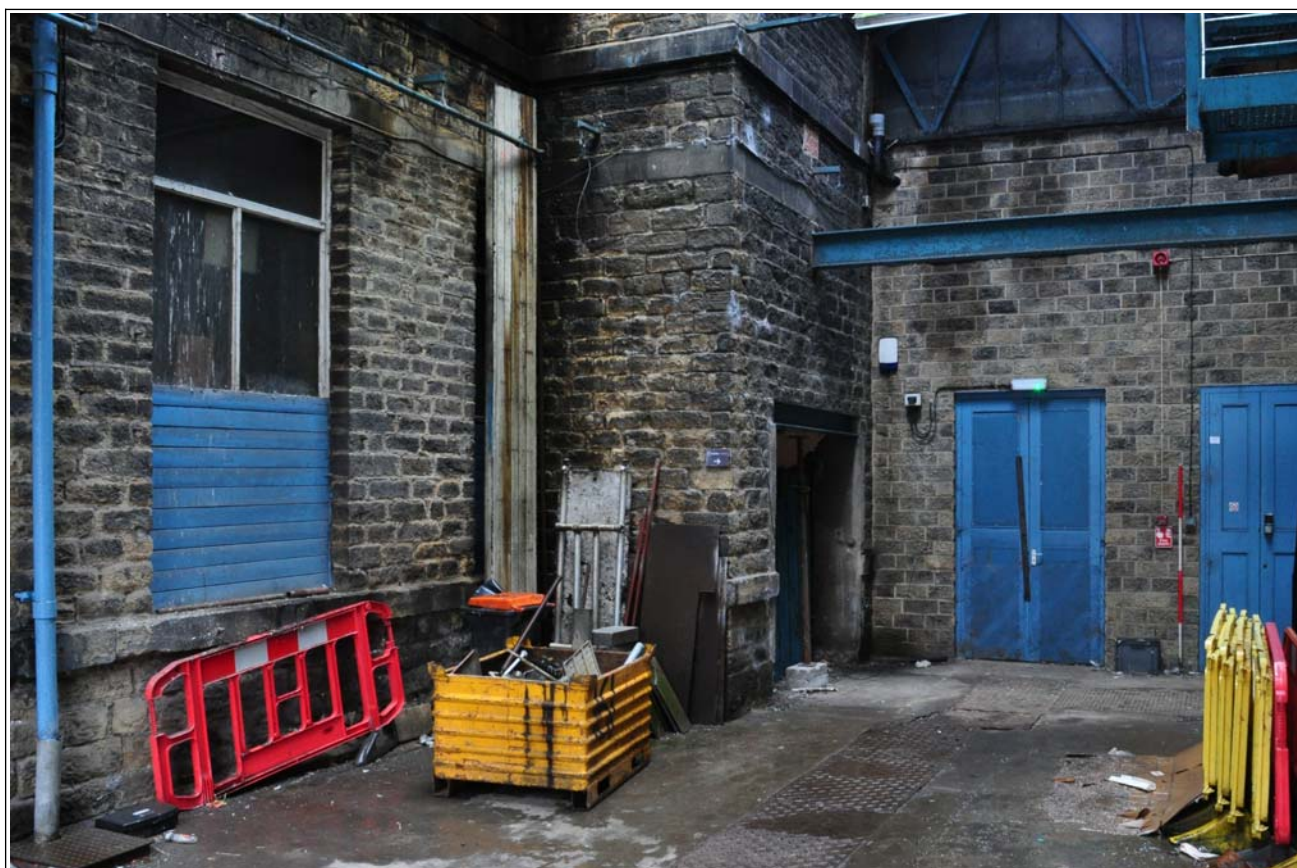
08: Building B (spinning block): foot of shaft/lift tower in south elevation
