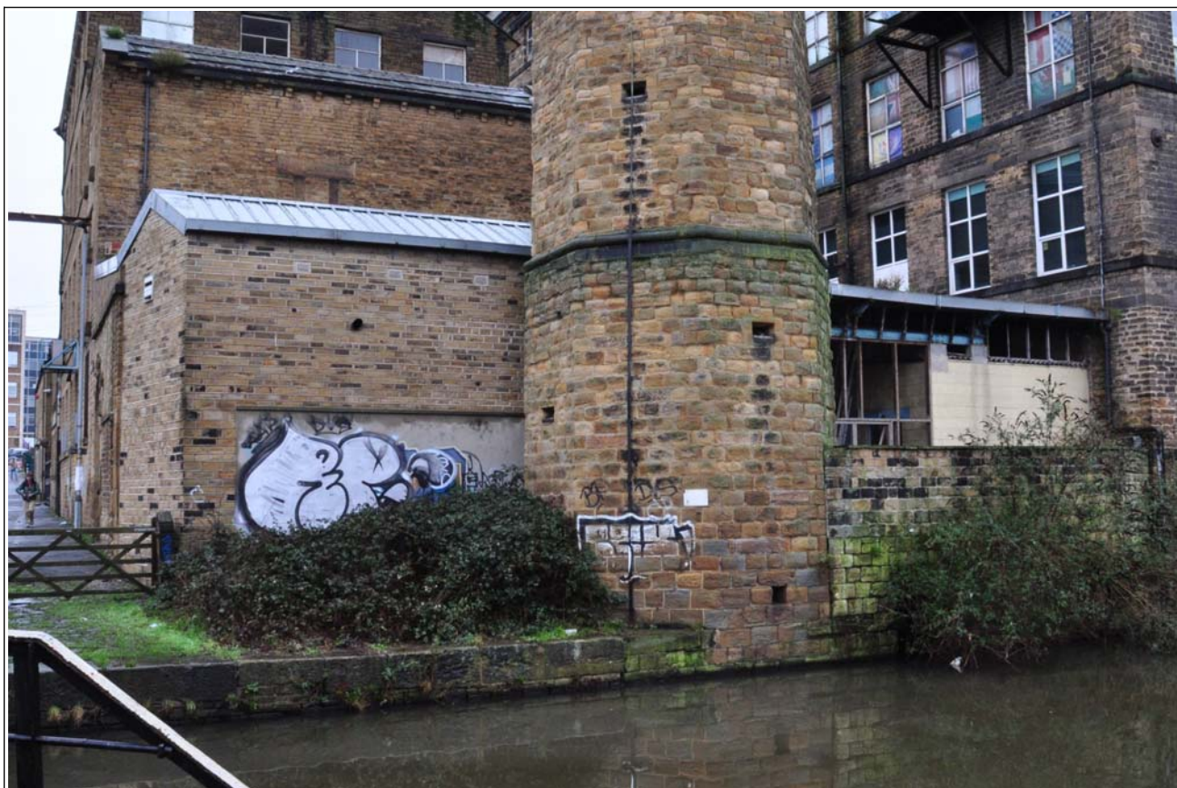
59: Building C (boiler house), looking west across canal, showing re-built part
