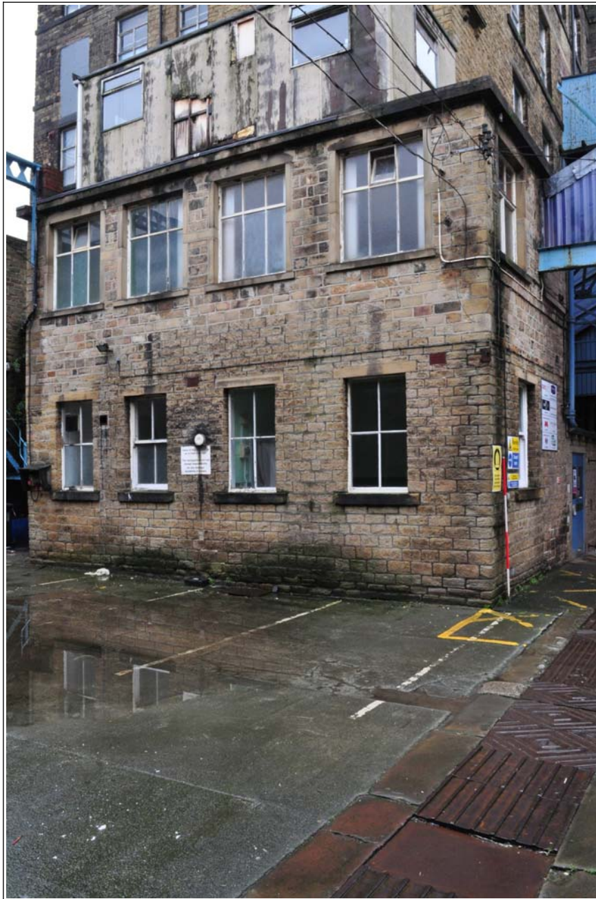
17: Building B (spinning block): extension on west side of stair tower, of ca. 1900 and later
