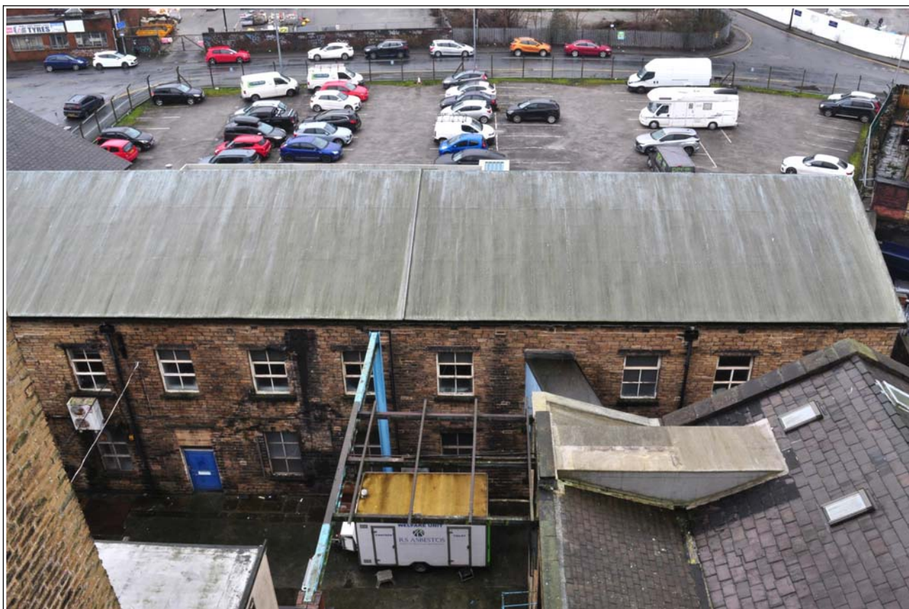
70: Building E (mill/warehouse), looking west
