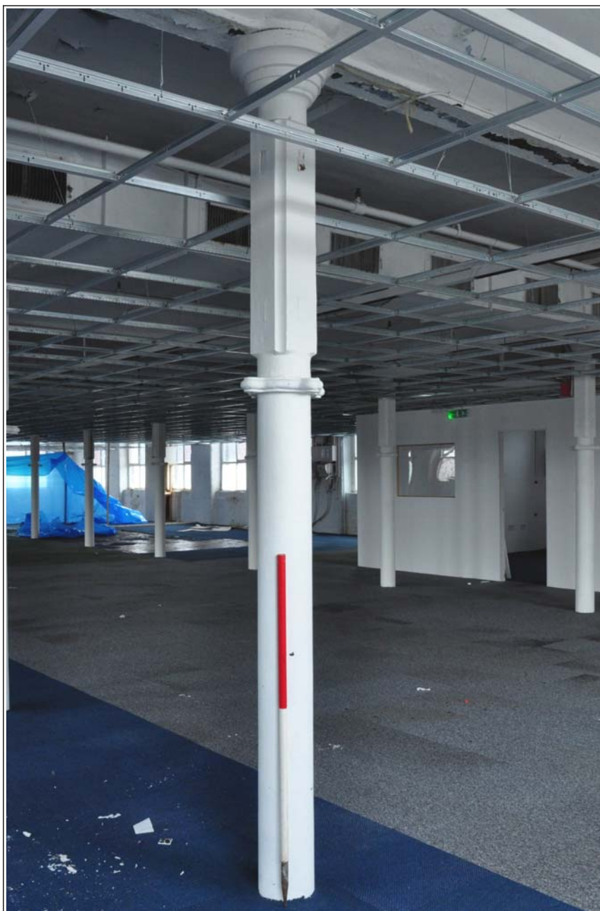
32: Building B (spinning block): typical column on fourth floor, looking south-east
