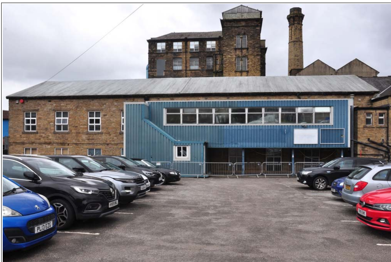
71: Building E (mill/warehouse), looking east, with modern WCs at right
