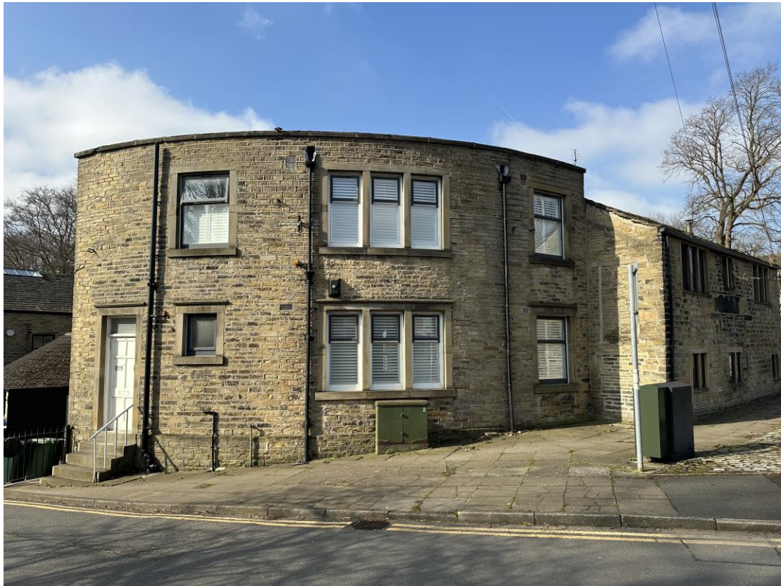
Photograph 1 – Elevation fronting the road
