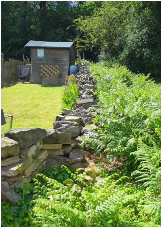
Figure 2: showing the low dry-stone wall.
