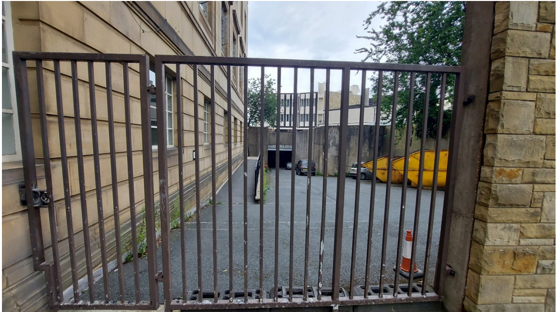
Plate 26: The sunken area to the east of the Library and Art Gallery with modern retaining walls and access to service tunnel.
