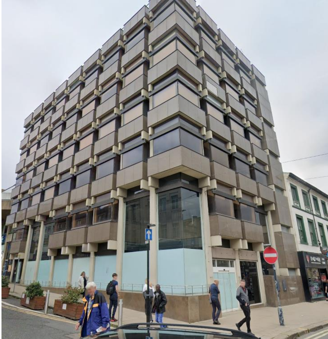
Photograph 2 – Entrance to the Upper Floors of Pearl House
