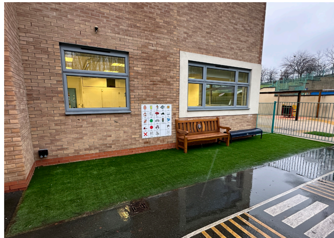
Existing Photo showing existing windows
