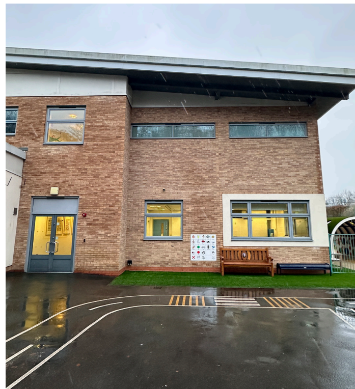
Existing Photo showing elevation where works are being proposed
