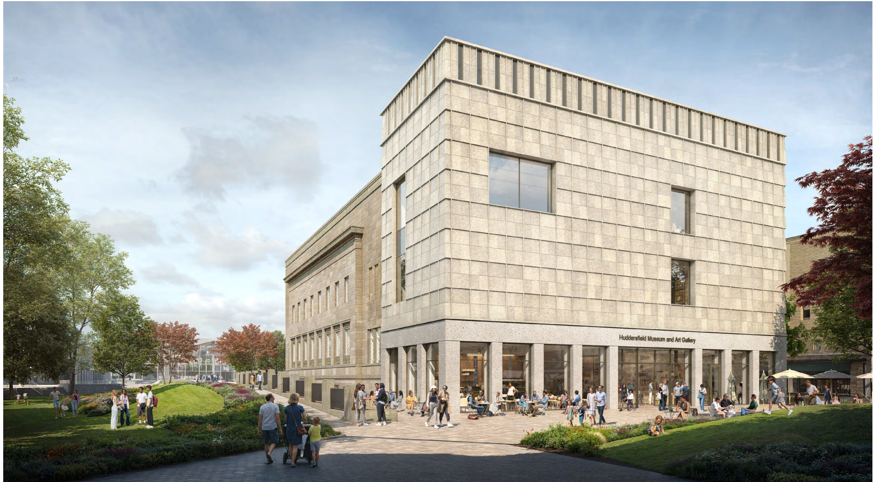
View from the Museum and Gallery North-East side, showing the new extension and entrance with existing fabric to east and Phase 1 in the background
