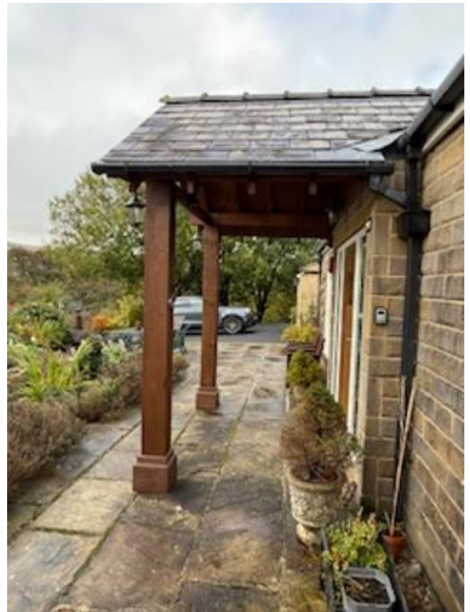
View of porch from the hall window
