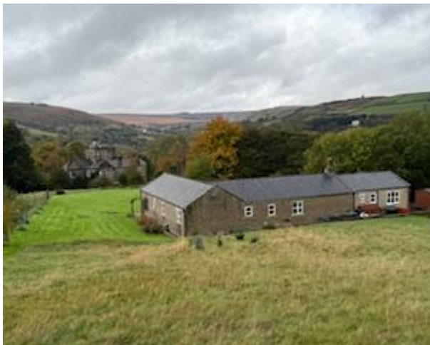
Rear elevation also showing property in front of our house (Crow Hill). The owners are happy with the proposal
