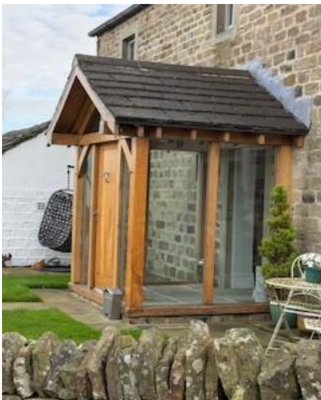
Similar type of design to our proposal though the door would be on the side
