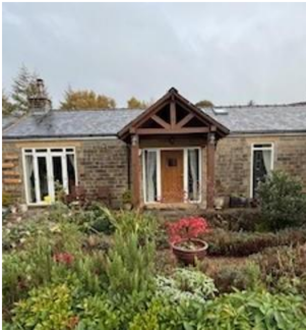
Front view of existing porch
