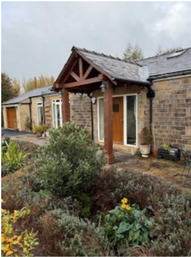
View of the porch from the bedroom window
