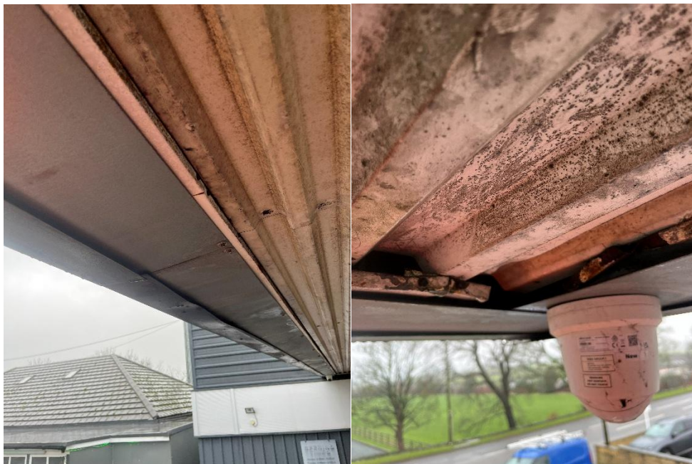
Plate 4: Gaps on the western aspect of Building B (left) and on the southeastern corner (right).
