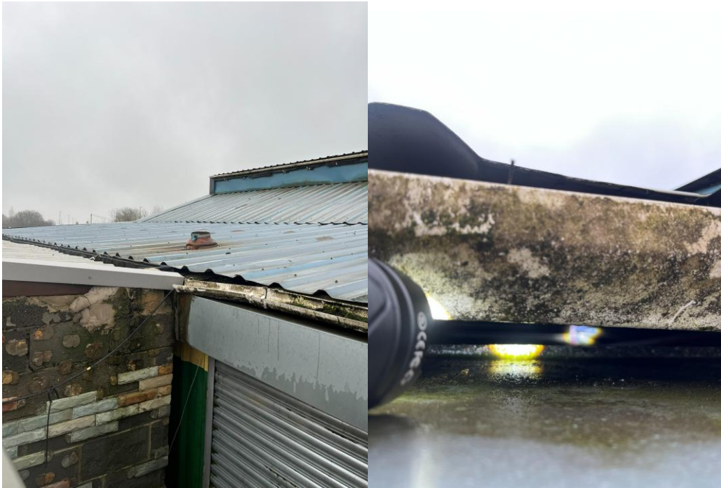
Plate 2: Showing the join between Buildings A and D (left) and resulting cavity (right).
