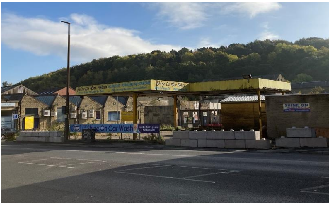
Figure 7.5 Ex Shine One car wash, Lockwood Road, Lockwood
