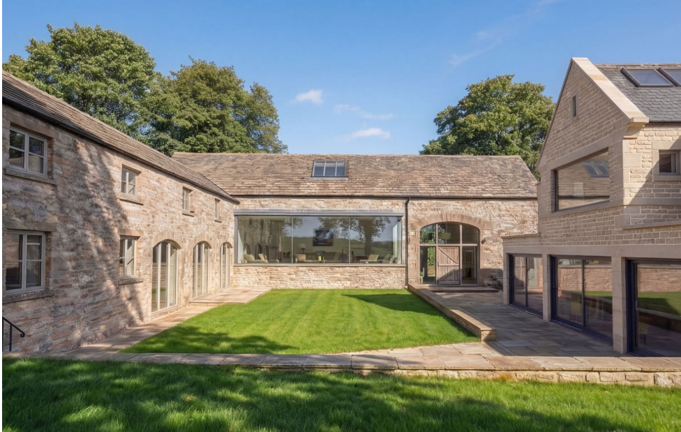
Illustrative View of the proposed scheme from the South East looking across the courtyard.
