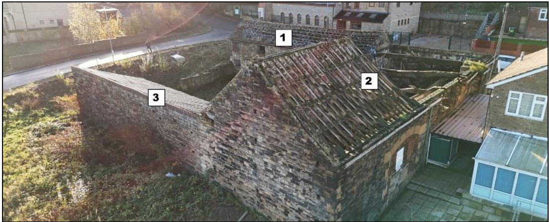
Plate 3. View of site from north with building sections numbered
