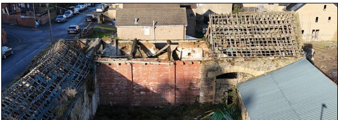
Plate 9. Southeast elevation of Building Section 2
