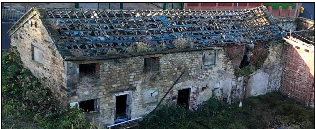
Plate 4. Building Section 1, viewed from east corner
