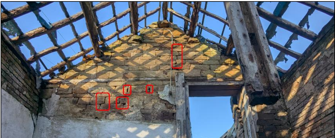
Plate 7. Crevices between wood lintel and masonry on Building Section 1
