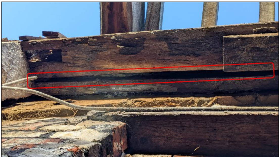
Plate 11. Crevice between lintels over double door opening in southeast elevation of Building Section 2
