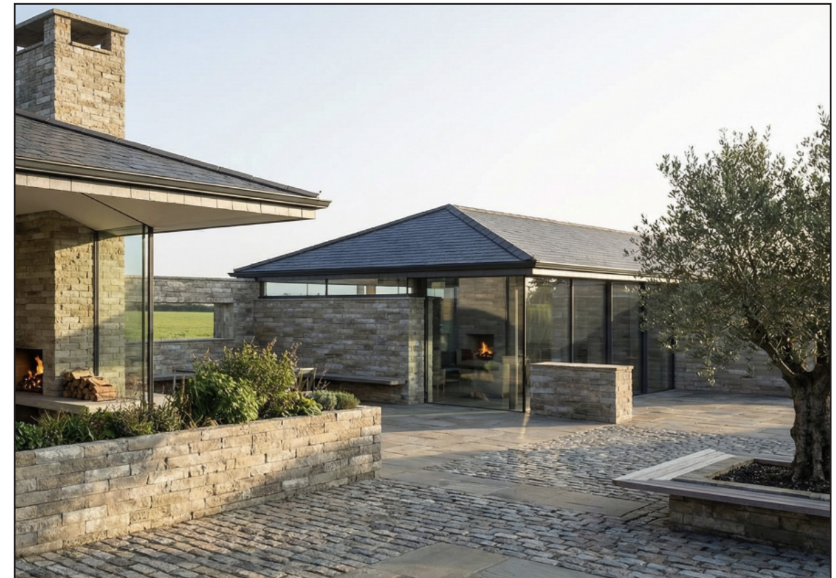
Image 08 - View towards the Courtyard / Fitness/Leisure Outbuilding
