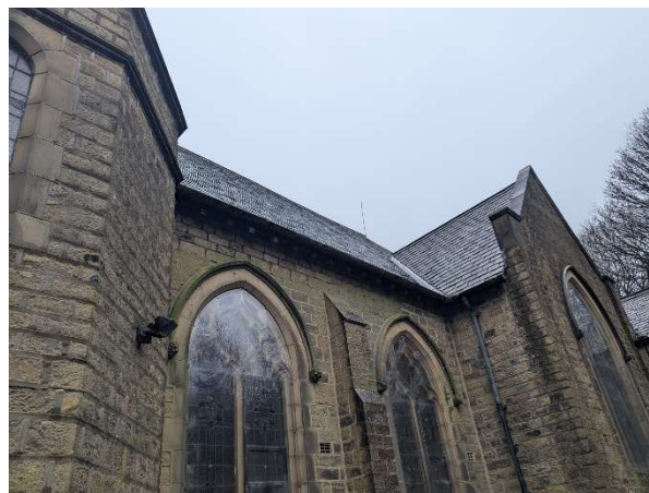
Photograph 5: Eastern aspect of the building.
