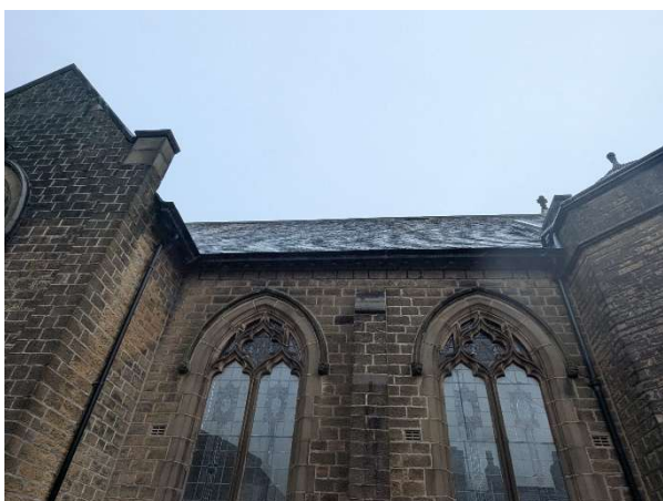
Photograph 3: Western aspect of the building.
