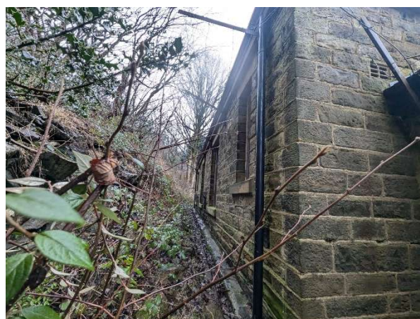
Photograph 6: Northern aspect of the building.
