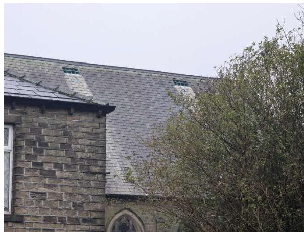
Photograph 4: Eastern aspect of the central pitched roof.
