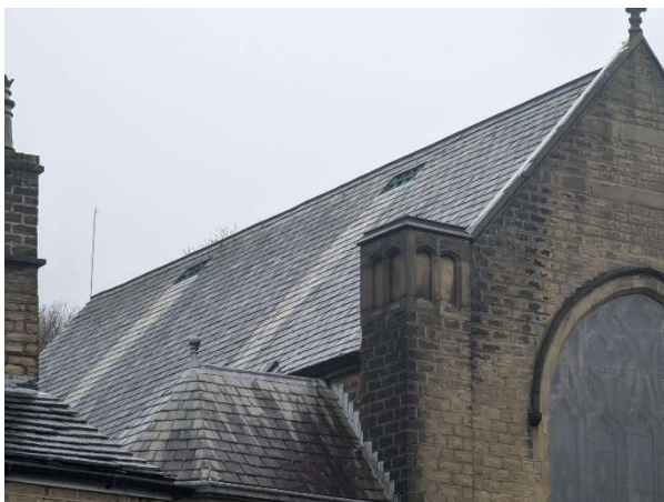
Photograph 2: Western aspect of the central pitched roof.
