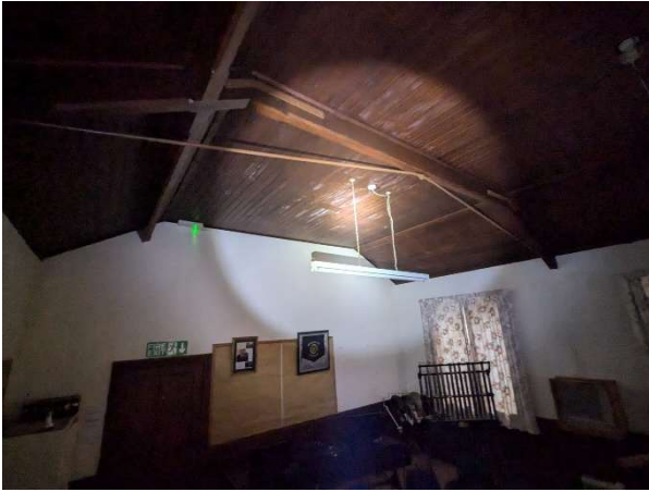
Photograph 13: Internal view of wood paneled vaulted ceiling.
