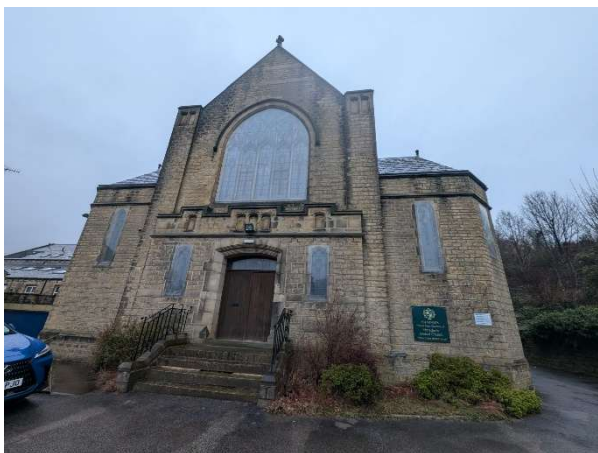
Photograph 1: Southern aspect/main entrance of United Church, Marsden.
