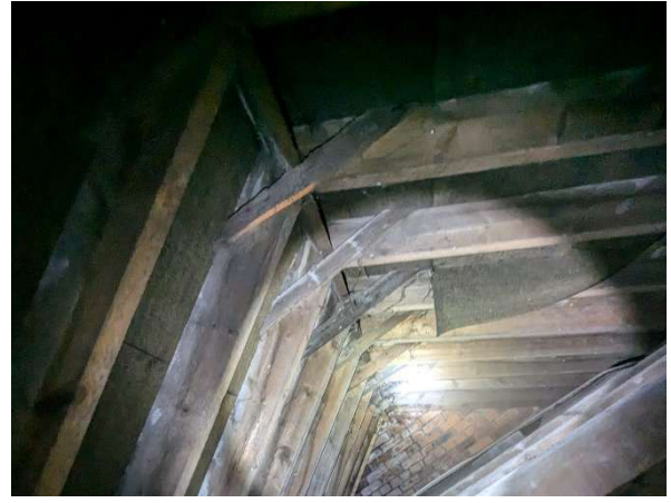
Photograph 16: Internal view of roof structure over a small loft space in the north of the building.
