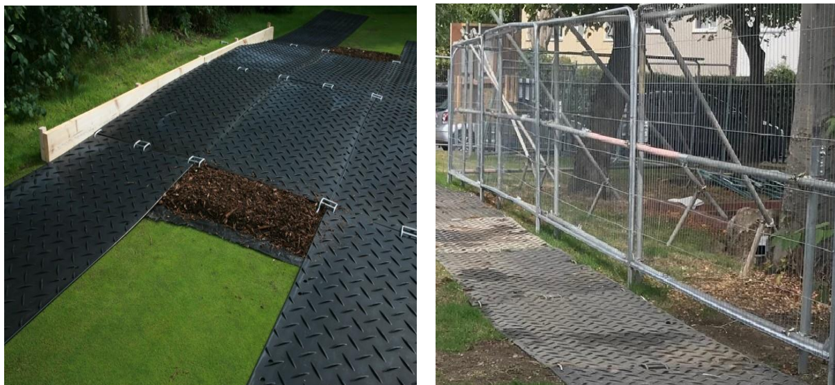
Figure 2 & 3. Examples of ground protection
