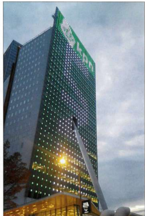
Picture 10.2: Digital media façade viewed locally, non-uniform light source
