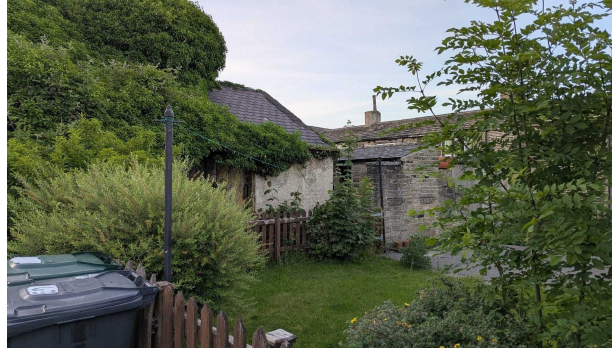
V1 B1-2 surveyor photo
