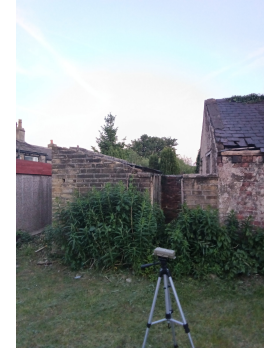
V1 B2-1 surveyor photo
