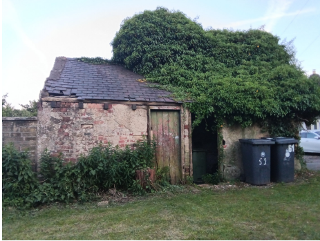
V1 B1-1 surveyor photo
