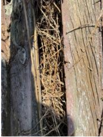
Photo 1: Dense ivy growth in room 4 preventing door from being opened
