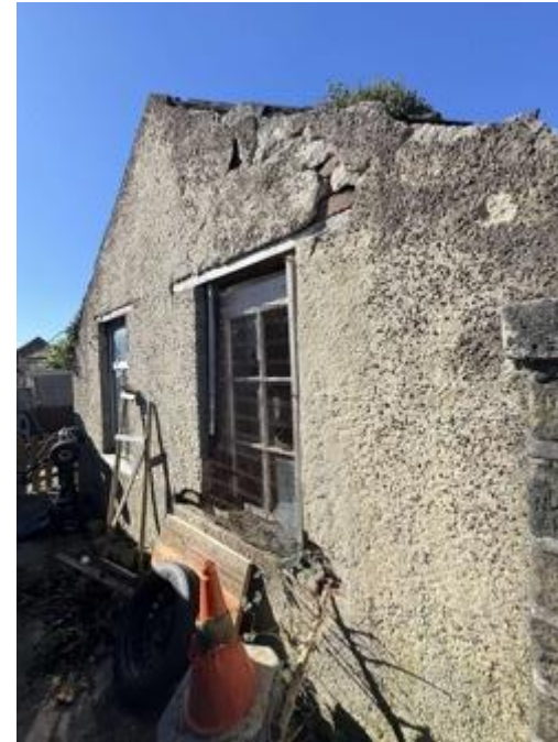
Eastern elevation of B1
