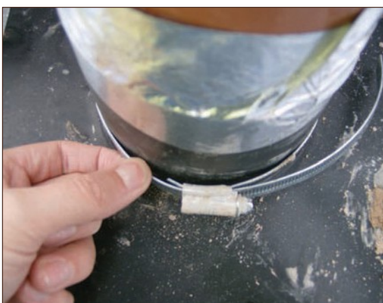
Figure A4.75 Jubilee clip on service entry insufficiently tightened so joint is uncompressed (courtesy Smith Grant)
