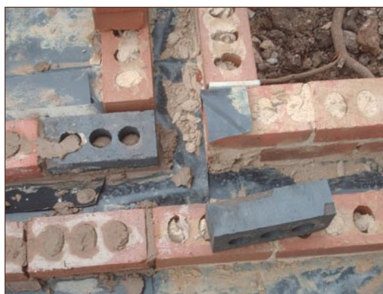
Figure A4.66 Follow-on trades proceeded work before gas membrane joints sealed (courtesy Card Geotechnics Limited)
