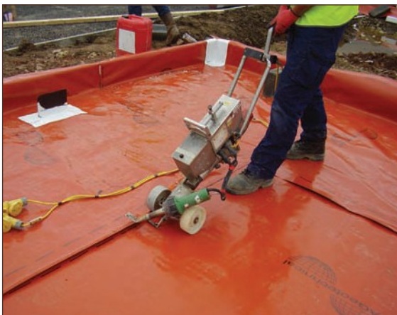
Figure A4.31 Extrusion welding (courtesy PAGeotechnical Ltd)
