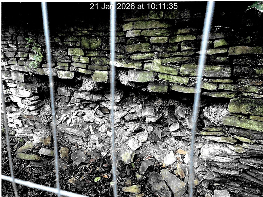
Wall collapse, poor masonry work evident in bonding.
