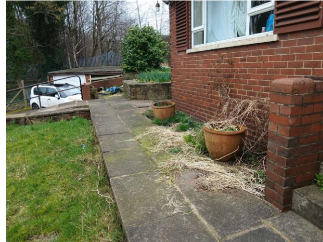
Photo 6: Paving around the main building
