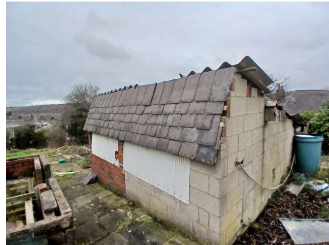
Photo 28: B6 - western elevation
