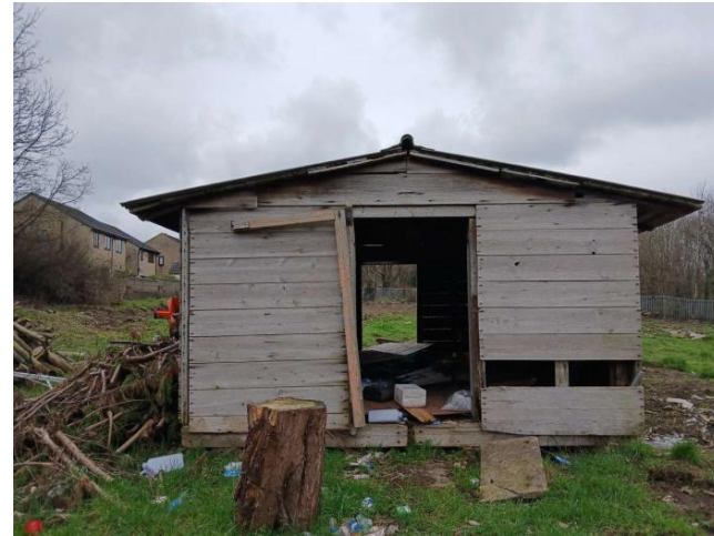
Photo 30: B7 - Eastern elevation
