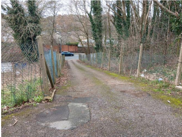
Photo 5: Tarmac access road
