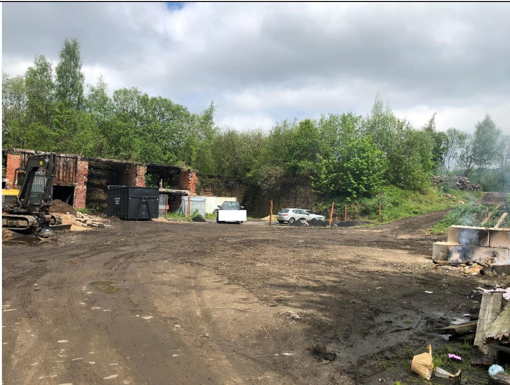
Figure 5: Photo taken in the south lower level of the site facing northeast. Coal drops noted to the left.
