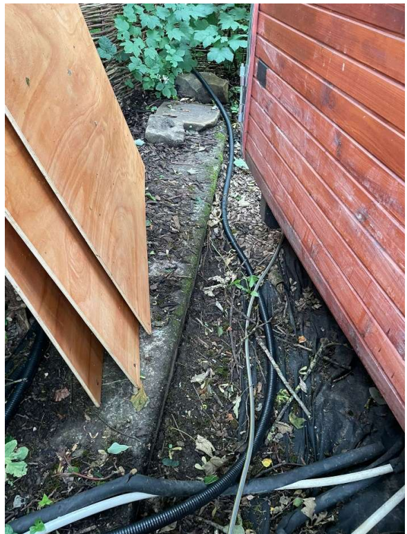
Photo 3 (left) plumbing on the plunge pools. Photo 4 (right) flexible hose route through the site.
