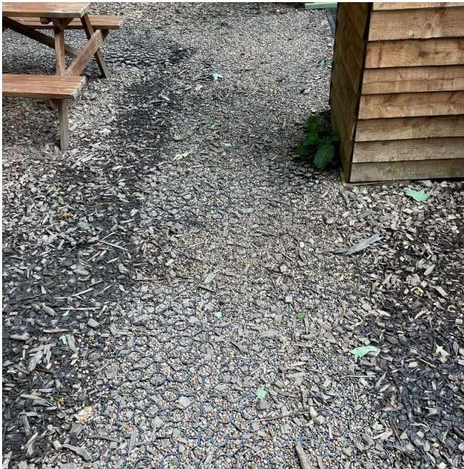
Photo 1 - Permeable floor surface through-out.
