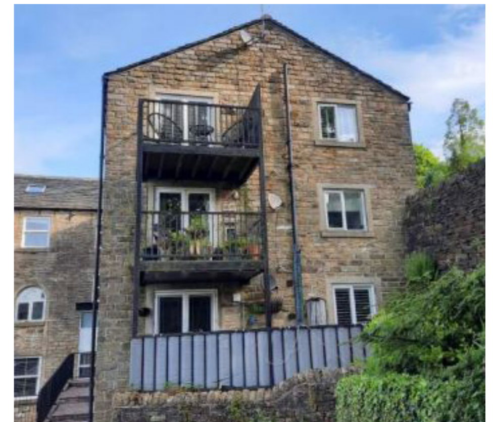
South Elevation - 116 Underbank.
