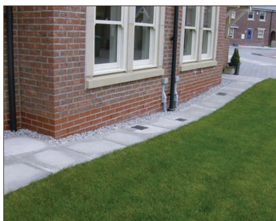
Figure A4.36 Raised air bricks are preferable due to the reduced potential for blockade but the vent trench specified is provided with clean single sized stone (courtesy Smith Grant)
