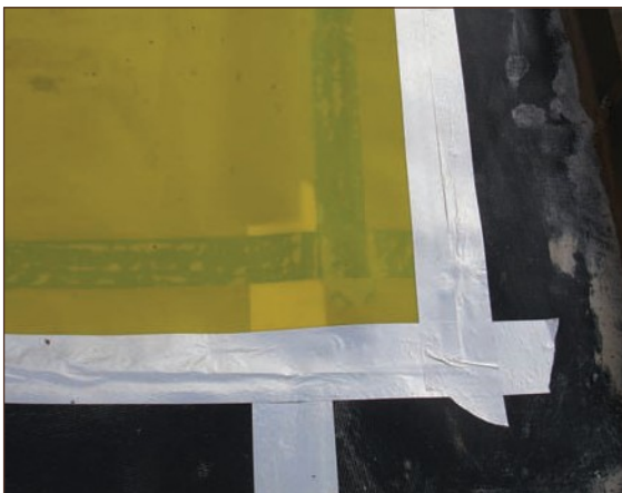
Figure A4.19 Well-constructed joints with gas resistant DPC, lap and double sided butyl joints visible beneath semi-transparent gas membrane, secondary seal with proprietary single sided tape (courtesy Smith Grant)
