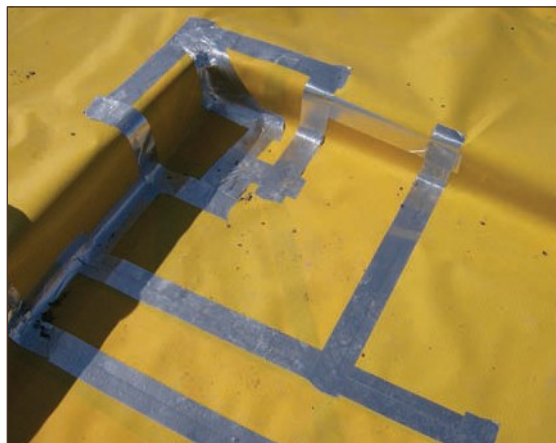
Figure A4.20 A pre-formed corner unit would have been preferable as fewer joints would have been formed, however the installer has achieved a good level of workmanship in this corner detail (courtesy Smith Grant)
