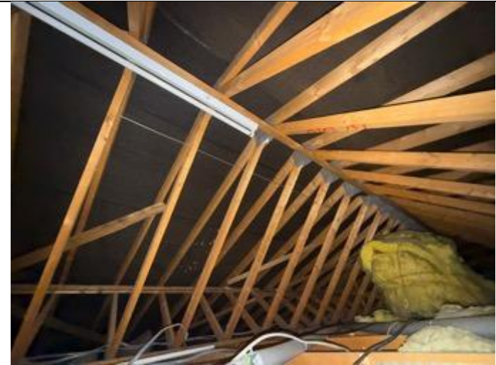
Roof space within B1
