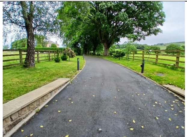
Photo 24: Access road with trees and vegetated garden parcels 4 and 5.
