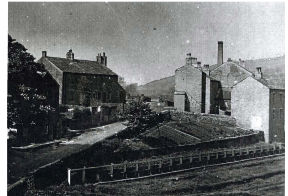
View of Warehouse Hill, Marsden in c1895 (Marsden History Group - www.marsdenphotoarchive.uk )
