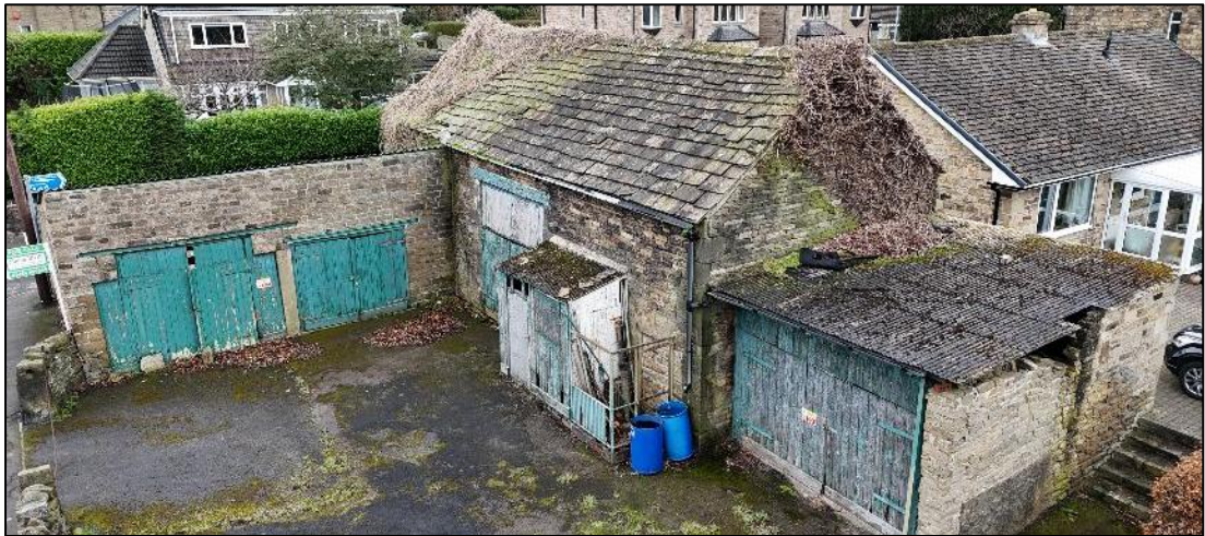
Plate 4. Building, viewed from south
