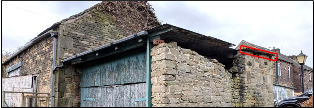
Plate 7. Access to wall top of single storey extension to northeast gable
