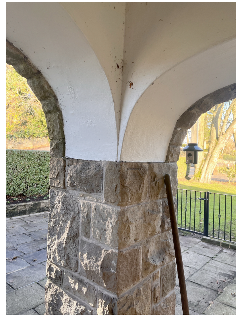
photo of existing stone to render detail
