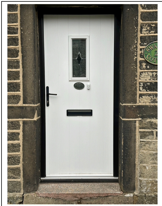
PHOTO OF REPLACEMENT DOOR
