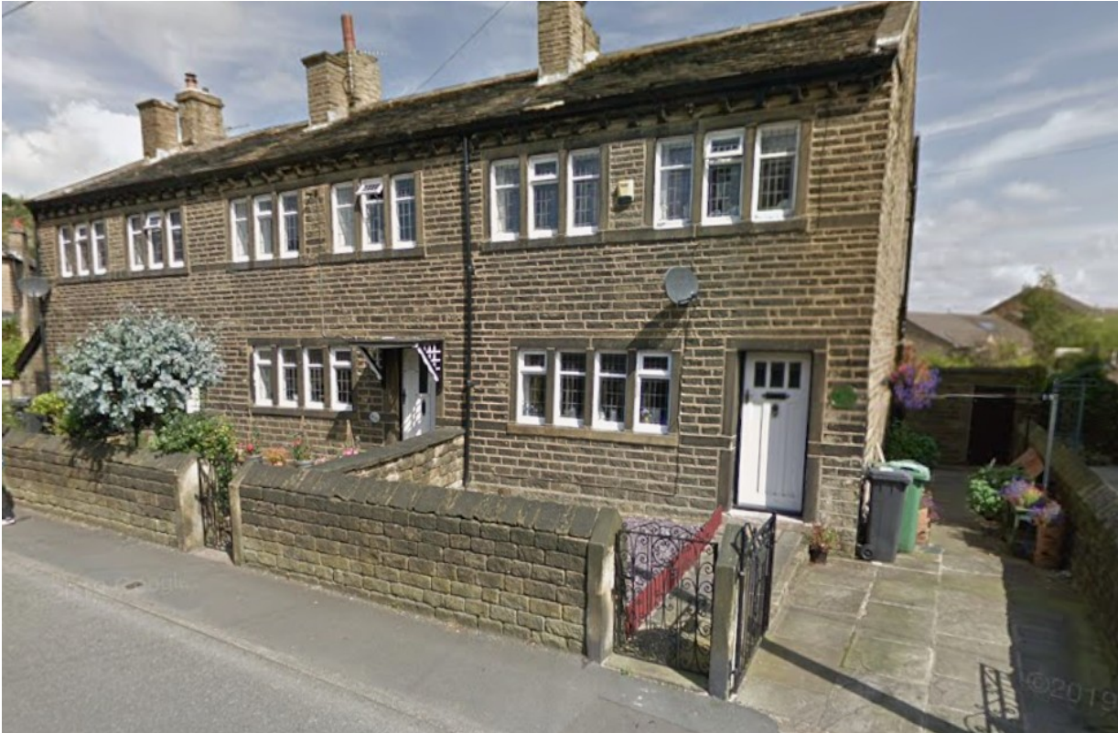
PHOTO OF ORIGINAL DOOR
