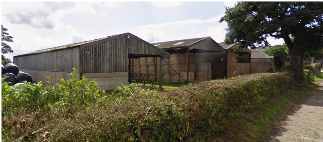
Field Lane (prior to new residential development) – vertical timber weatherboarding and corrugated roof
