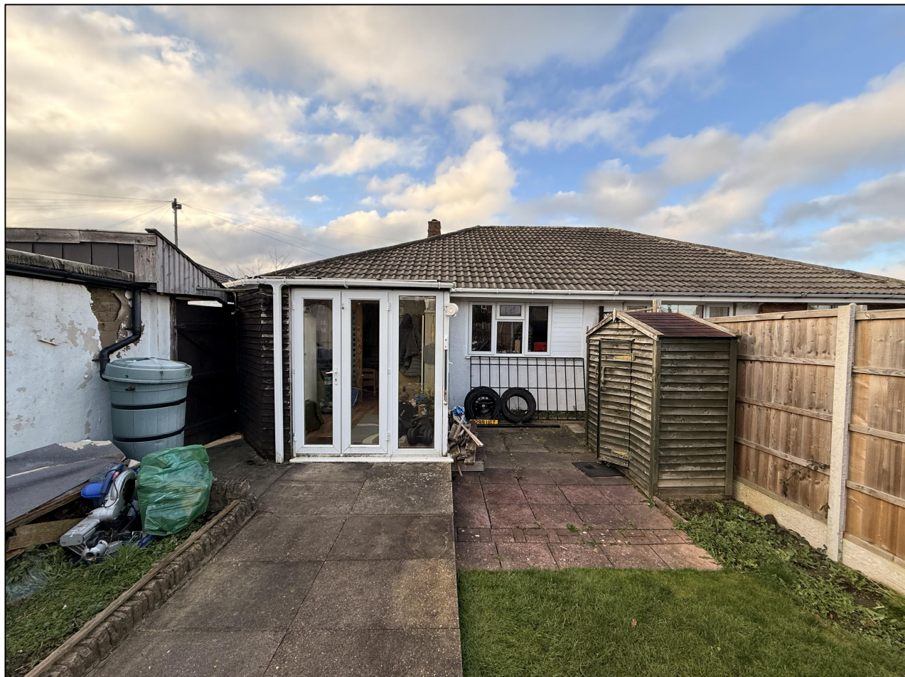
Existing rear elevation photo
