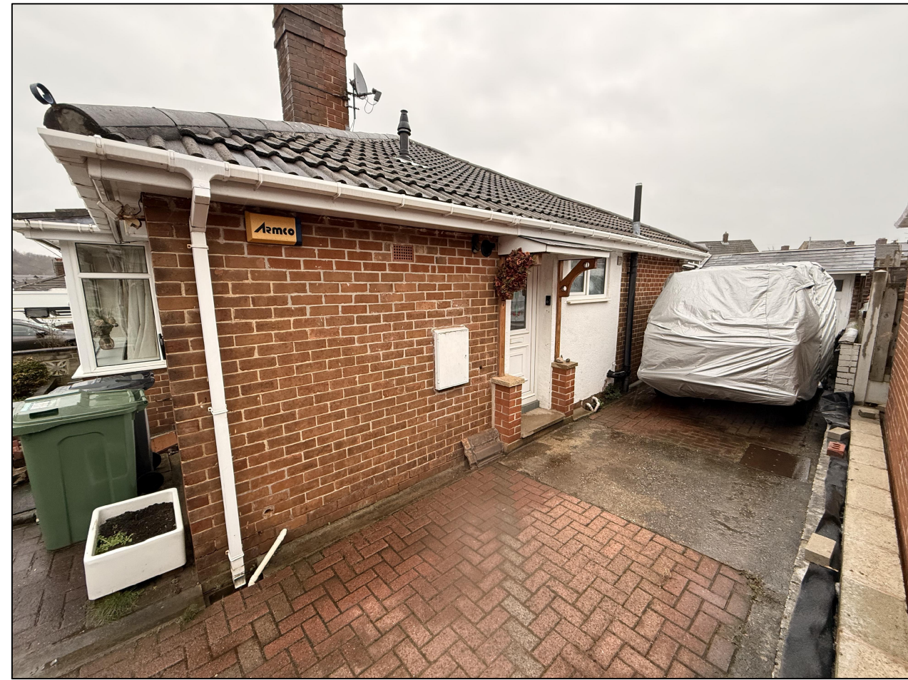
Existing side elevation photo
