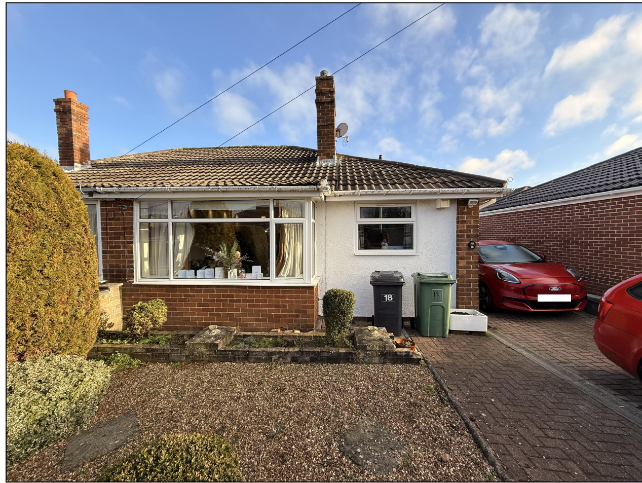
Existing front elevation photo
