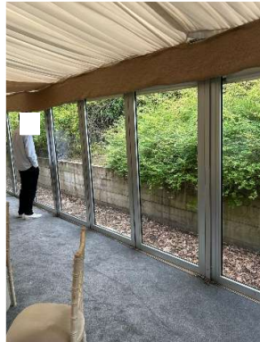
Above: existing interior view towards the rear of the site
