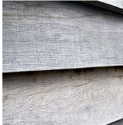
Timber Horizontal Boarding
