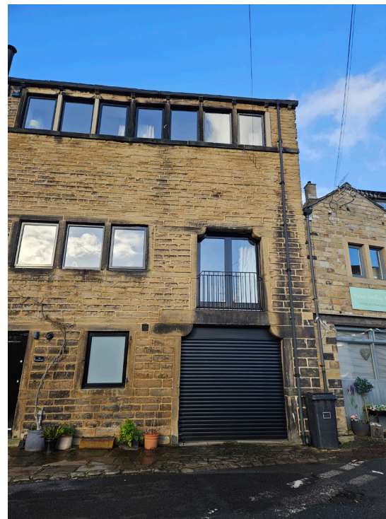
② Example of French doors and juliet balcony at 'The Warehouse' Old Road
