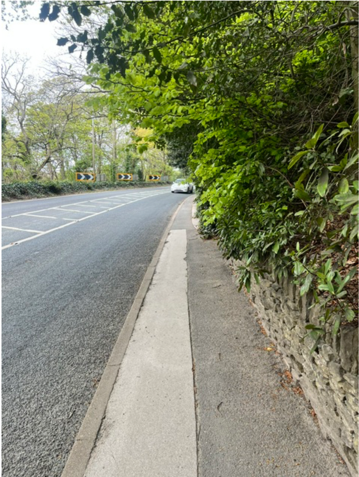
Photograph 2 – narrow footway, having to lean over, torso is at risk of being struck. Vehicles emerging at speed around blind bend. No streetlights.
