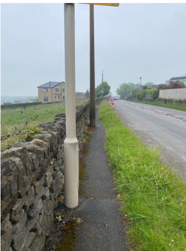
Photo 8: Narrow pavement with obstructions Barnsley Road
