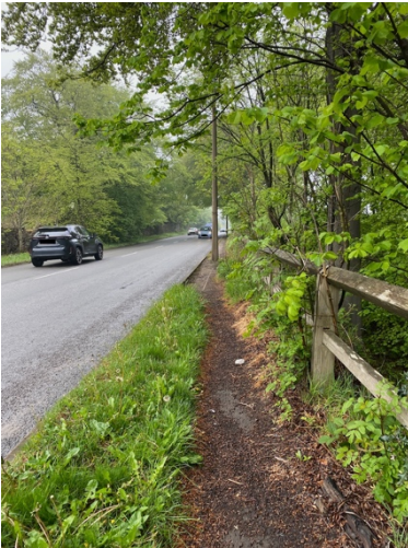
Photo 7: Barnsley Road pavement – lamp post obstruction
