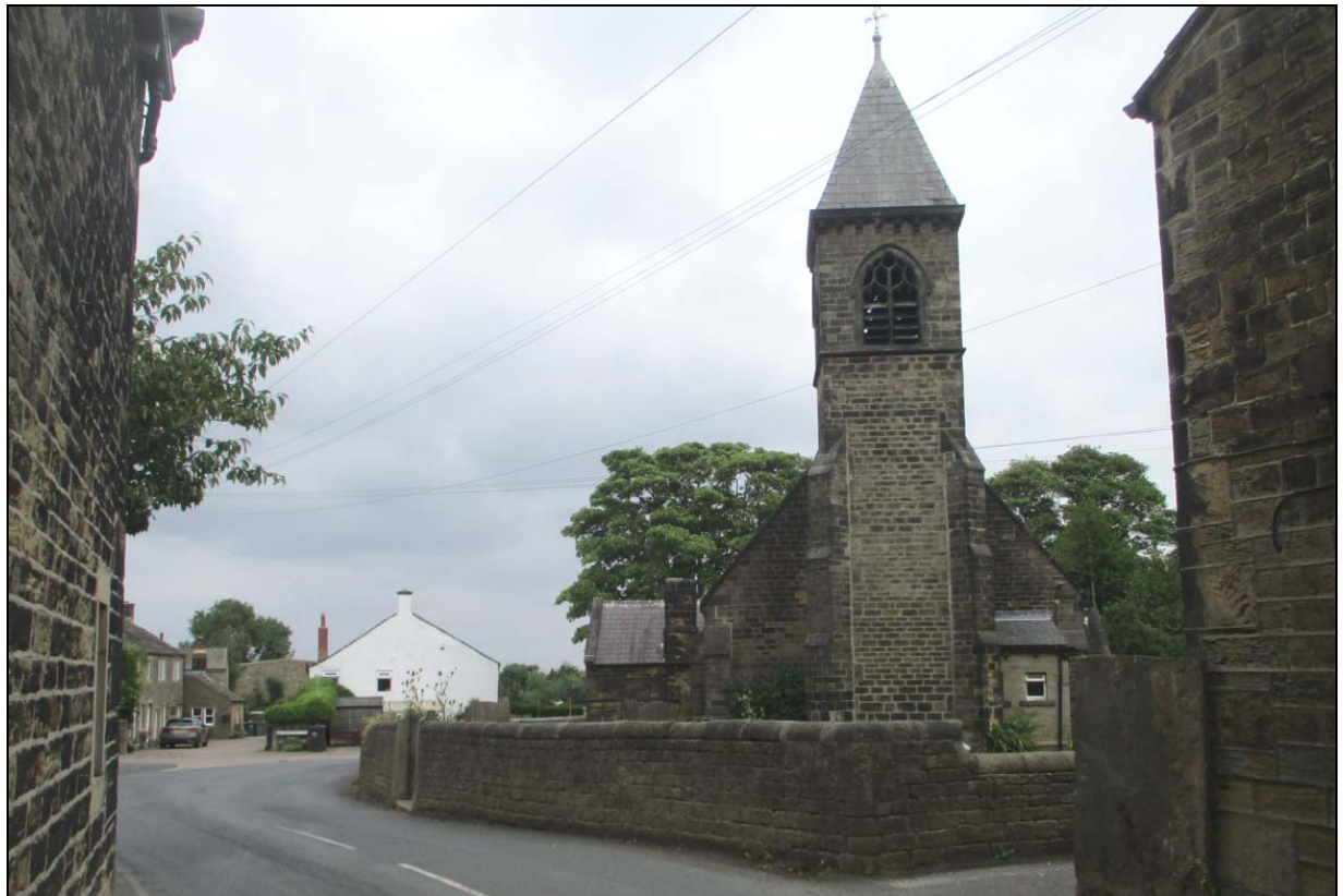
The clustered core of the conservation area is centred on St Nicholas' Church
