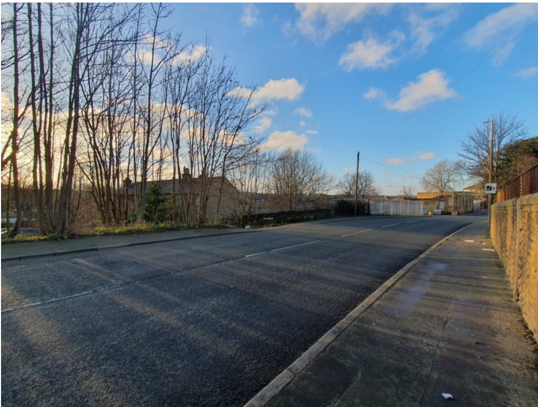
Above: View of existing wall to site B from Walkley Lane.
